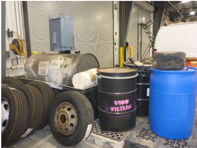
Photo 8: One 200-gallon tank containing used oil, one 55-gallon drum containing used oil filters, and one 55-gallon drum containing oil contaminated rags observed in the Transportation Department. The tank was labeled with the words “used oil”.
