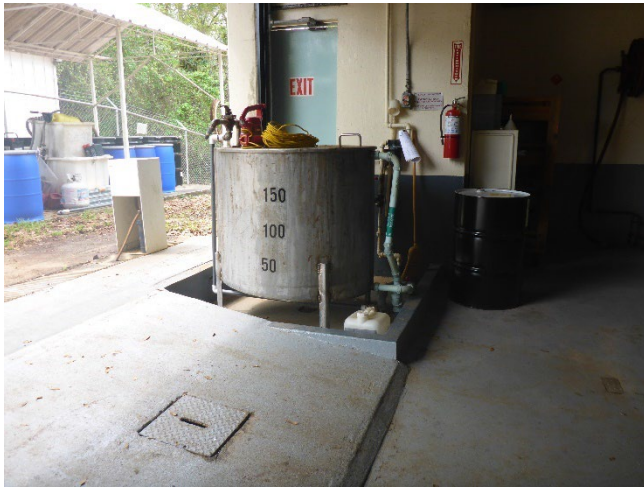
Photo 4: 250-gallon neutralization tank, which was empty at the time of the inspection.
