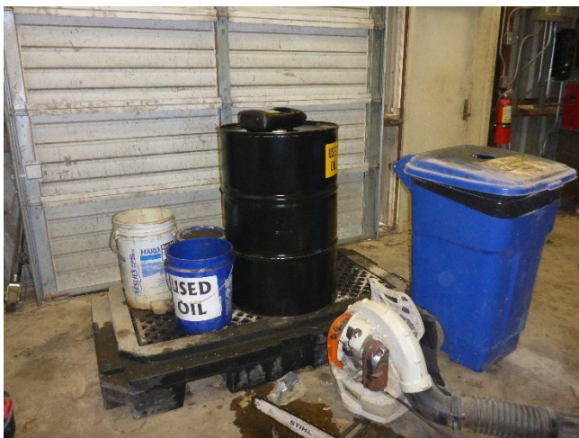
Photo 6: A secondary containment pallet holding one 55-gallon drum of used oil, one 5-gallon bucket containing an oil filter and absorbent material, one 10-gallon bucket containing oil contaminated rags and one 3-gallon container of sharpening compound observed next to a trash can containing oil contaminated rags in the Landscaping/Grounds Maintenance Area.
