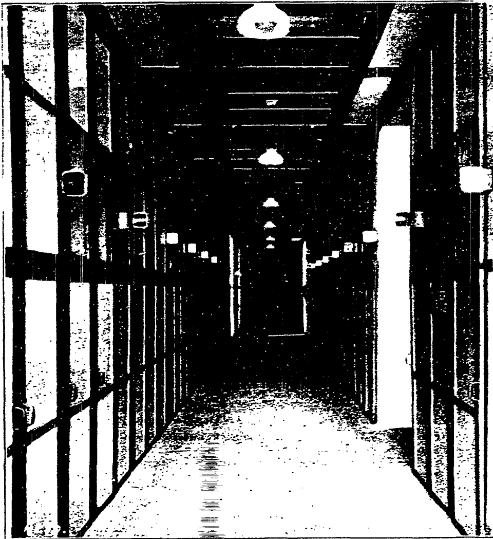
PL. 10. BUS SWITCH COMPARTMENTS
