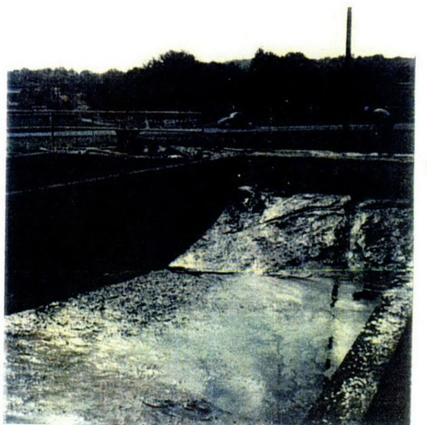
N. Pit showing third cascade looking East 6/21/77
