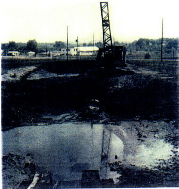
N. Pit from inlet toward dike. 6/21/77
