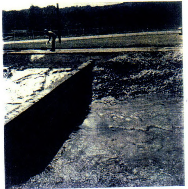
N. Pit mid cascade during cleaning 6/21/77
