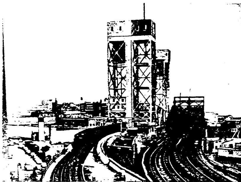
Soon to replace altogether the older bridge at right is the New York Central Railroad's twin-span lift bridge over the Harlem River in New York City. Like its predecessor, the new bridge depends upon red lead for first line protection against corrosion.
