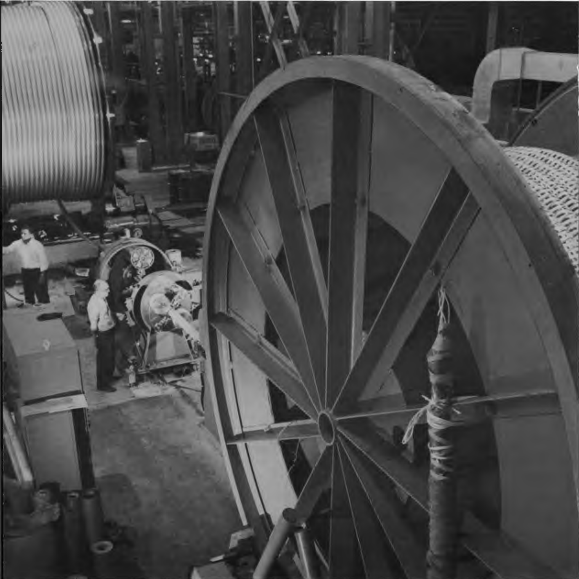
A 345,000-volt cable passes between mammoth 14-foot reels at Okonite's Paterson, N. J. plant as the final D-wire is applied. These reels, designed specifically for use with extra high voltage cable, can accommodate 3500 feet of four-inch diameter cable.
