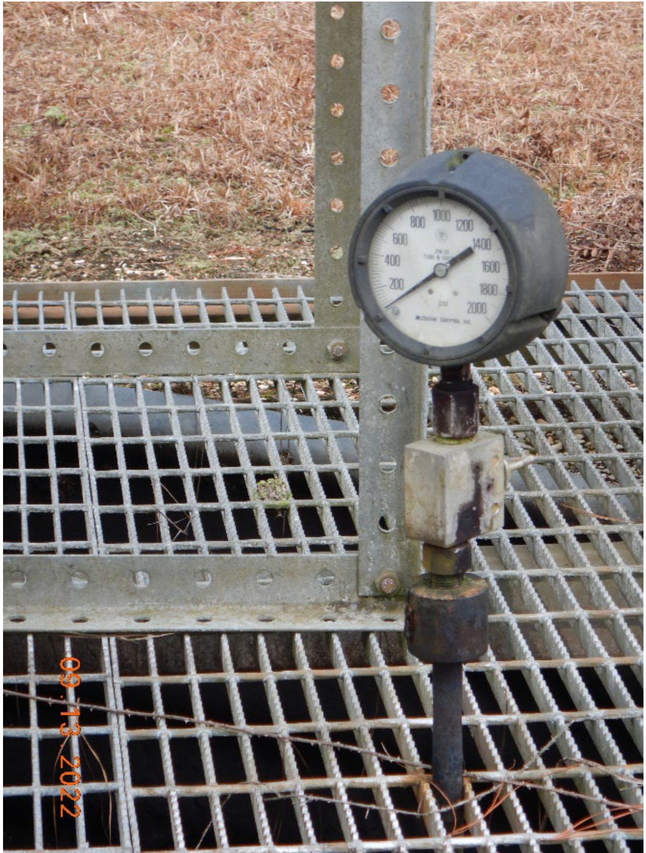
Photograph 2: Looking west, closeup view of surface pressure gauge reading 0 psi.
