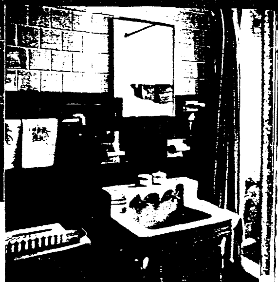
Porcelain-on-aluminum wall tile is easily installed and presents an attractive finish as shown at right. Lead compounds are an essential ingredient of the porcelain.
