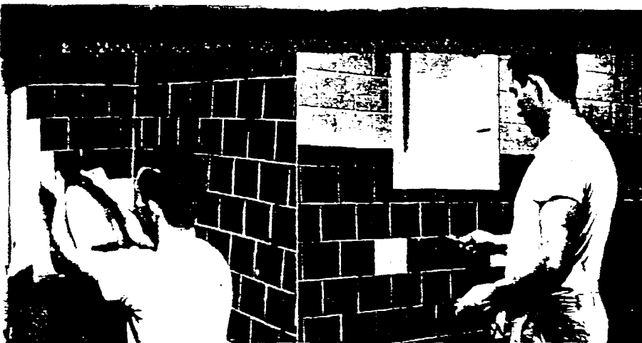
Porcelain-on-aluminum wall tile is easily installed and presents an attractive finish as shown at right. Lead compounds are an essential ingredient of the porcelain.
