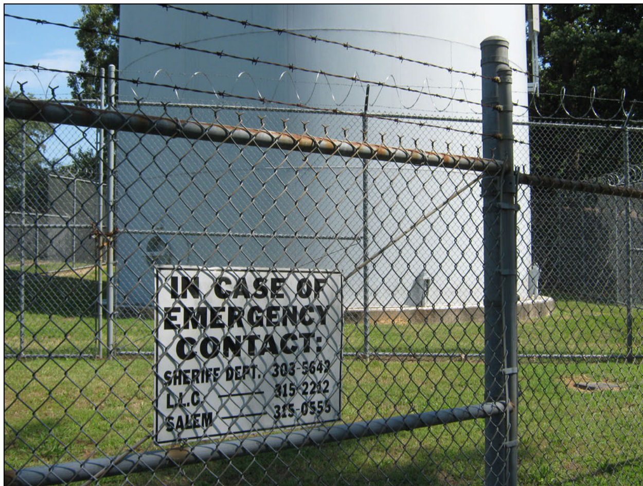
Photograph 9. Mulberry/Salem Tank View of an emergency contact sign that was prominently attached to the outer fence at the Mulberry/Salem Tank. A “No Trespassing” sign was not present.
