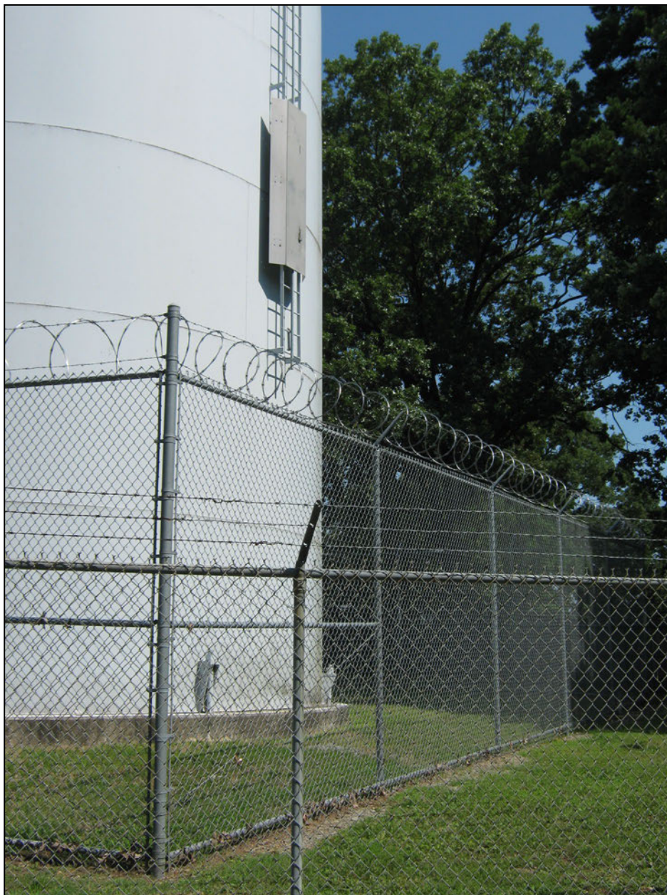
Photograph 8. Mulberry/Salem Tank View of the double-fence system with the innermost fence equipped with razor wire and access ladder modified to above ground level.
