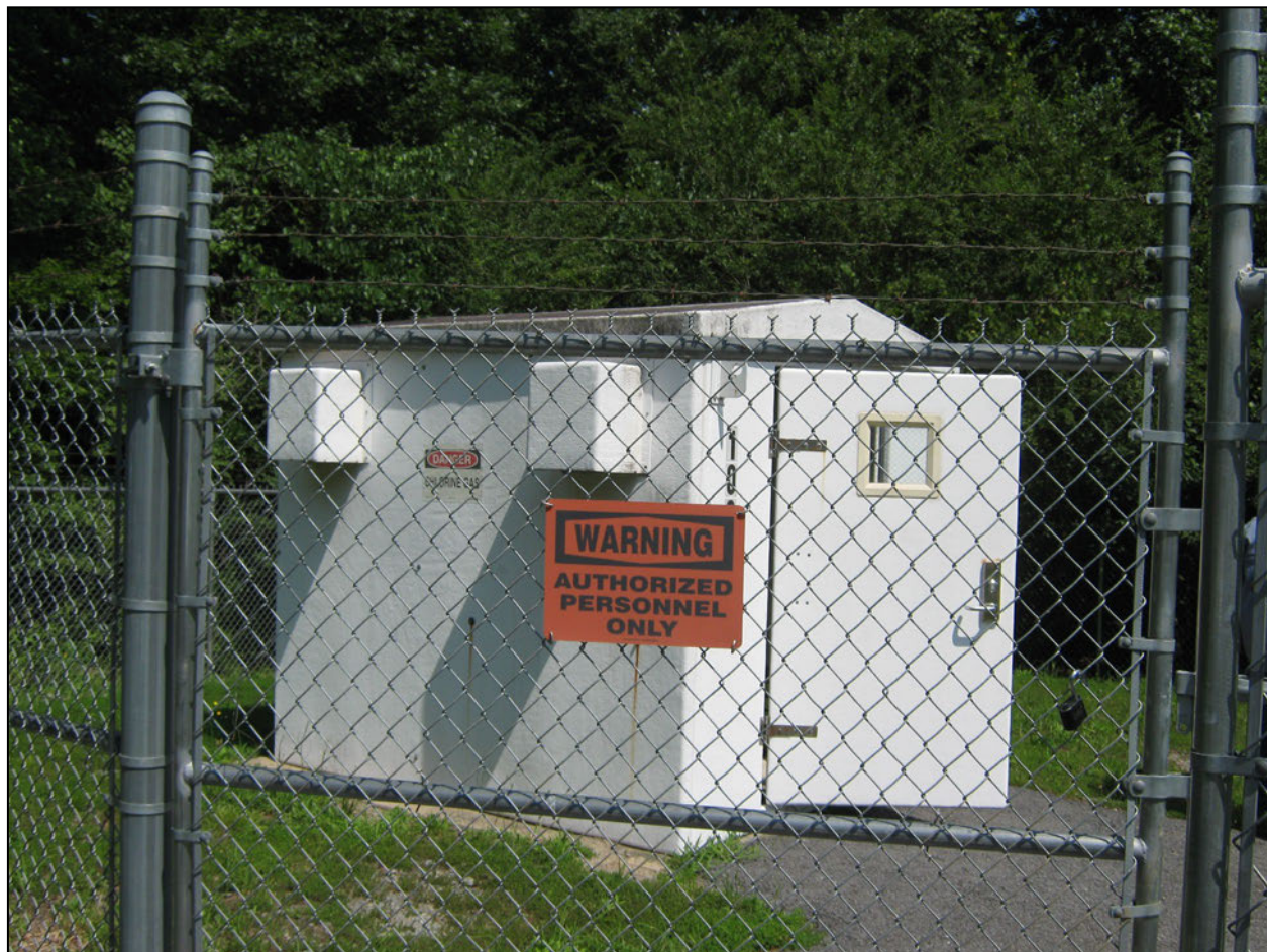
Photograph 13. Sparks Chlorine Booster Station View of the exterior of the chlorine storage and chlorine feed entrance door. A distinct second room had a rear entrance door (not in the photograph view).
