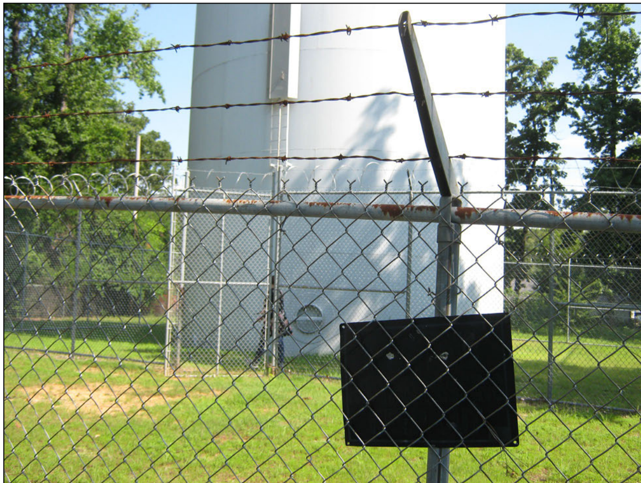
Photograph 1. Longhills Tank View of the double-fence system with the innermost fence equipped with razor wire and access ladder modified to above ground level. The “No Trespassing” signage was unreadable.
