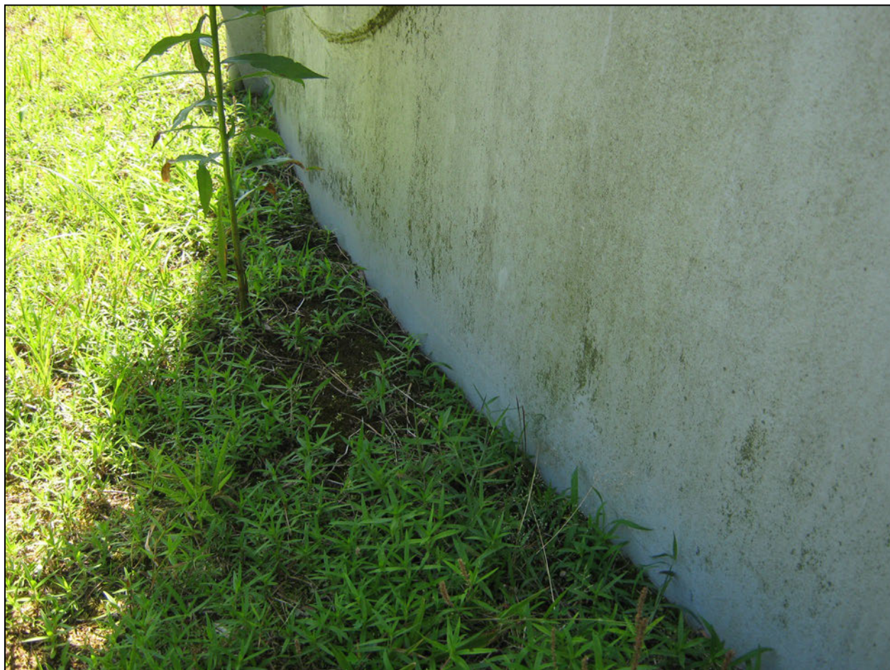
Photograph 7. Longhills Tank View of the concrete base of the Longhills Tank that was covered with soil above the base seal and to the sidewall of the tank.
