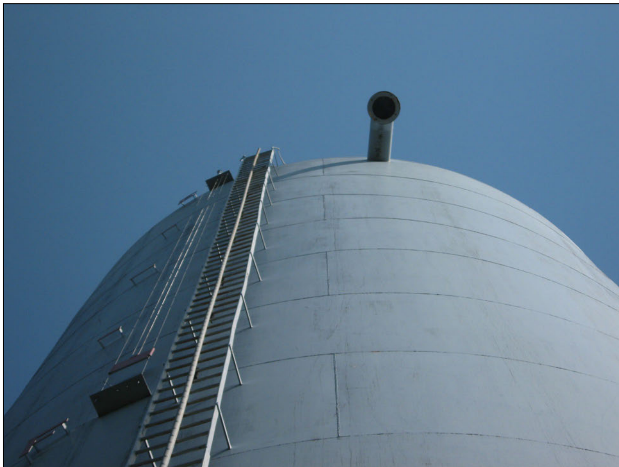
Photograph 4. Longhills Tank Alternate view of the Longhills Tank overflow. The overflow was downturned but did not extend to ground level. The overflow did not allow for evaluation for adequate screening.
