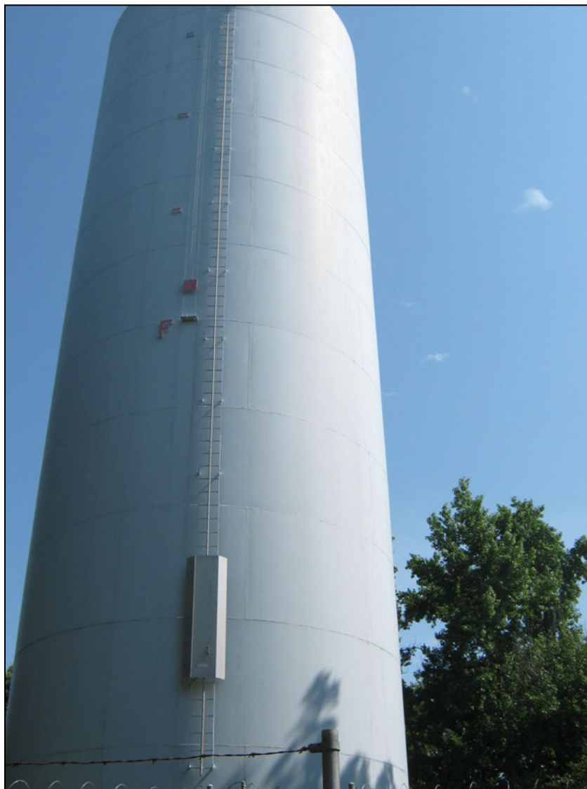
Photograph 2. Longhills Tank View of the Longhills Tank access ladder that was cut above ground level and shielded with a ladder guard.
