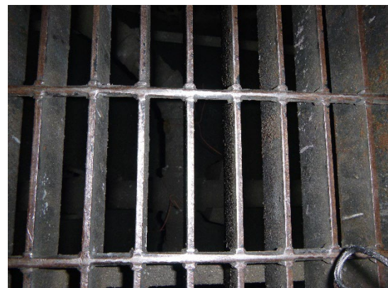
Photograph 6: Hazardous waste piping from Return and Fill Station boxes.
