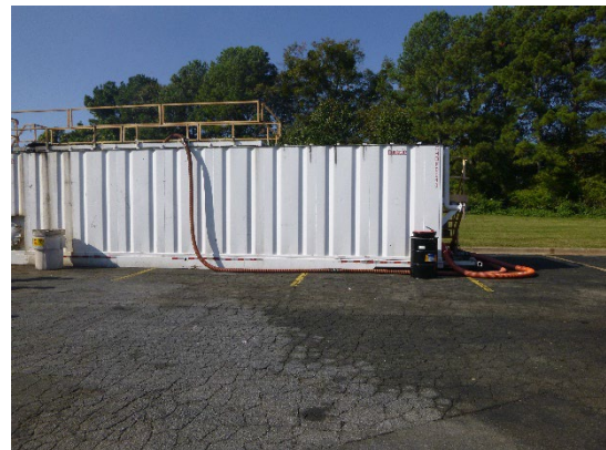
Photograph 18: Frac Tank in parking lot.
