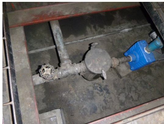
Photograph 8: Tagged filter and pump under grate in Fill and Return Station.
