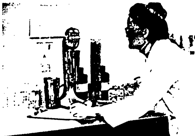
Hydrometer analysis of soils.
