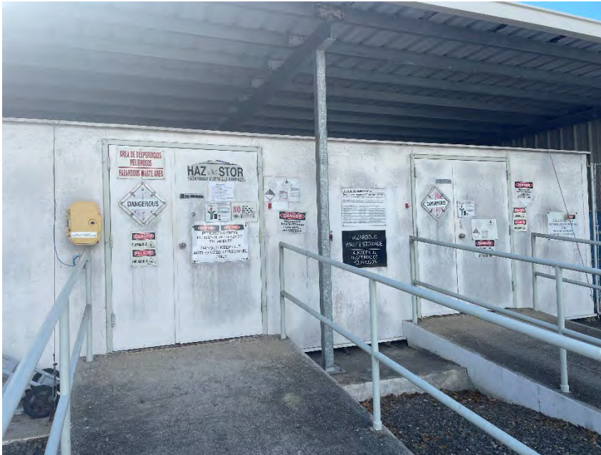
Photograph Five (5): Outside overview of the CAA PR1.
