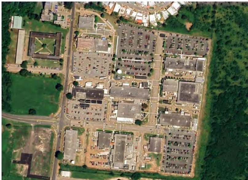
Figure 1: Overview of Hamilton Sundstrand de Puerto Rico, Inc. Aerial Photograph
