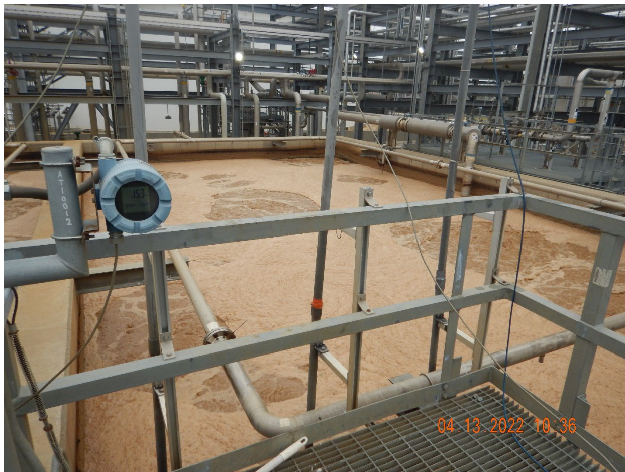
Aeration Basin A.
