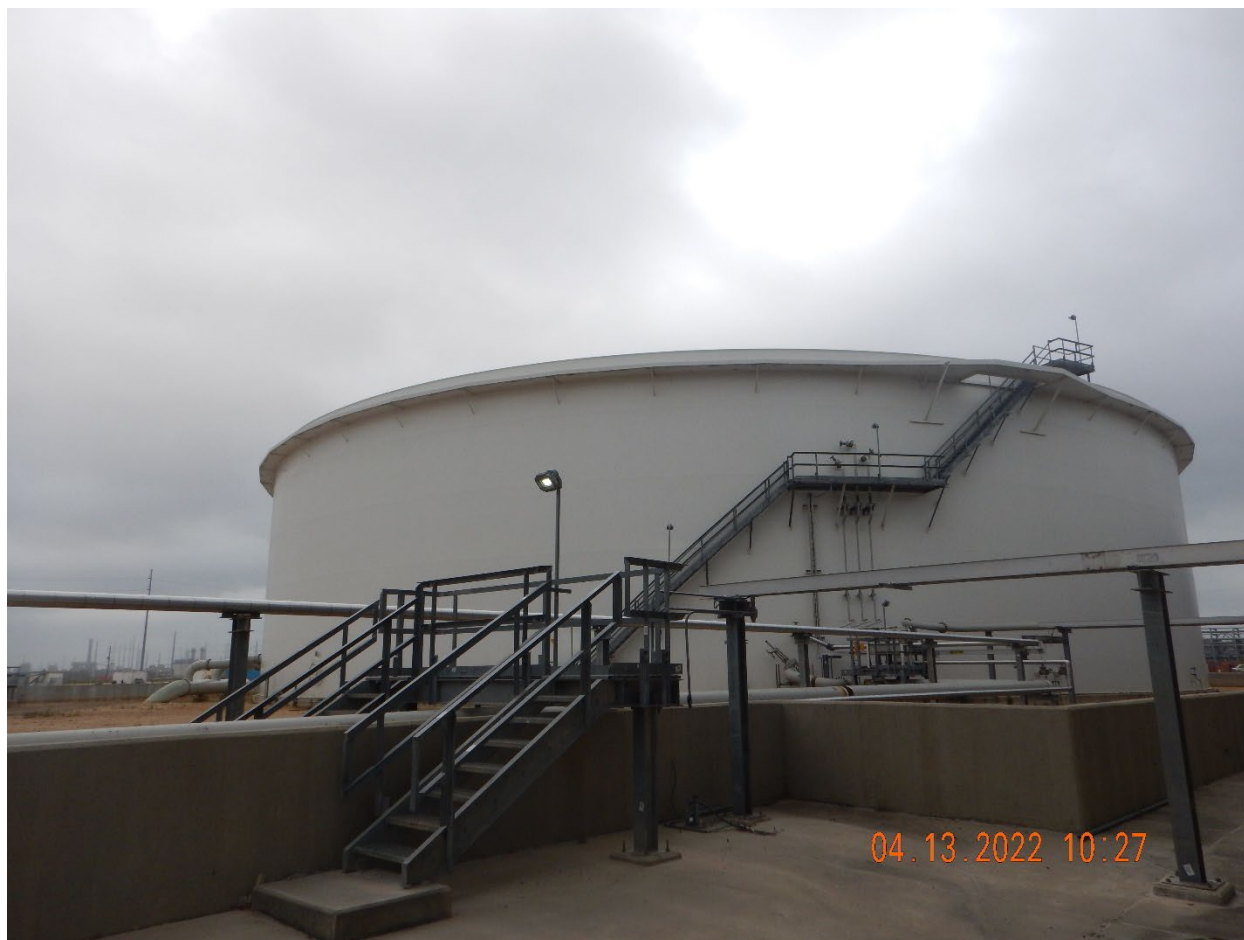
Storm Water Tank.
