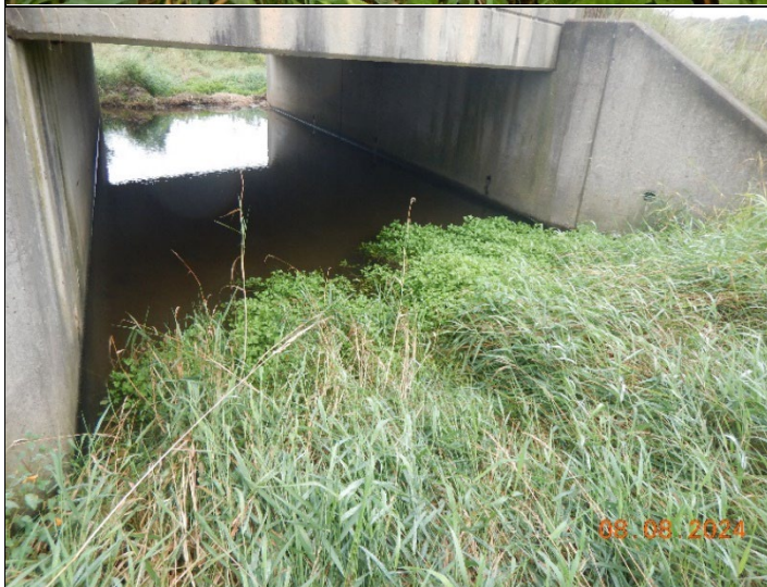
Hoopes Property Date: 8 August 2024 Photo ID: DSCN5581.JPG Photo taken by: Laura Mathew Notes: Downstream view of the Genessee River flowing into culvert under Loucks Mill Road.
