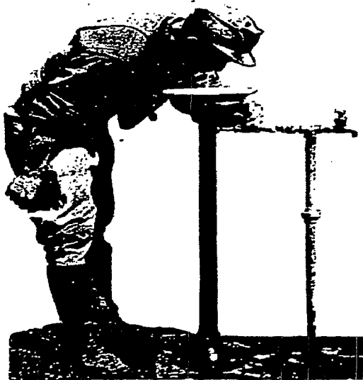
Drinking fountain faucet at entrance to mine. Jet of water is delivered at an angle.
