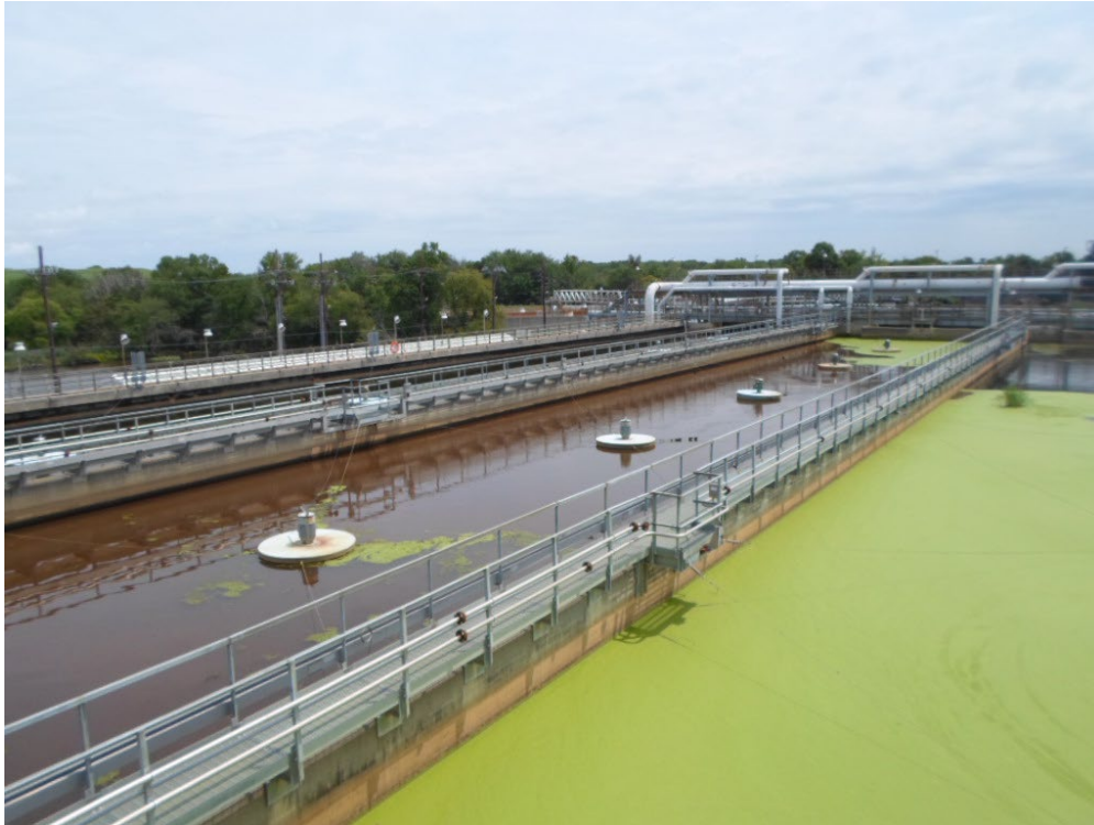
Photograph 33. Duck weed covering approximately 10% of Cell B (center of image) of tertiary aerator AE-251 at the WWTP.
