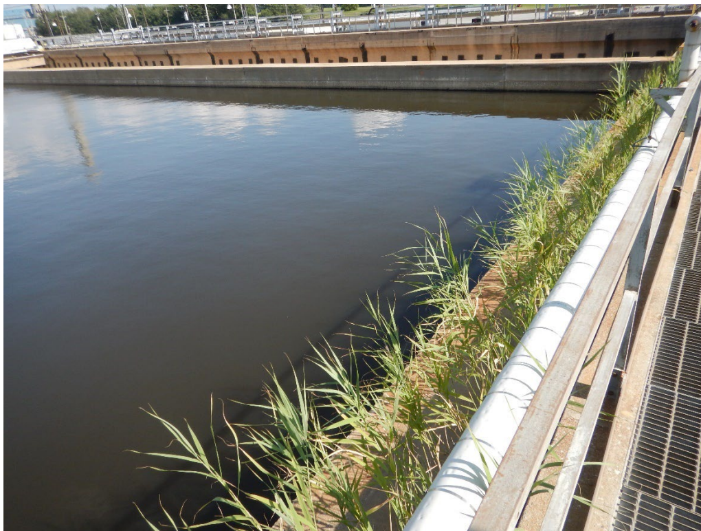
Photograph 26. Vegetation along the primary clarifier CF-63 at the WWTP.
