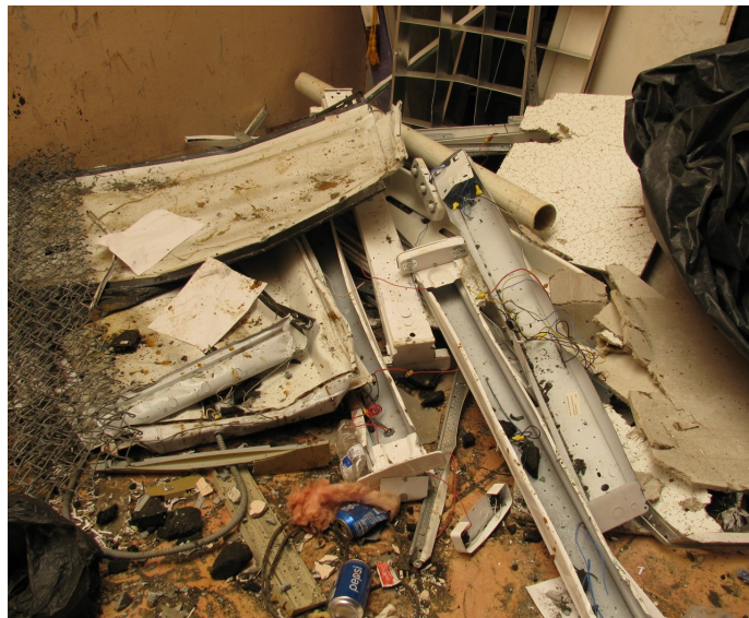
Picture 2 - CHARLES HARDWOOD MEMORIAL COMPLEX, ST. CROIX- At the Main Building Entrance Area, there were various broken fluorescent lamps on the floor mixed with aluminum frames and ballasts without control or containment of Universal Wastes.
