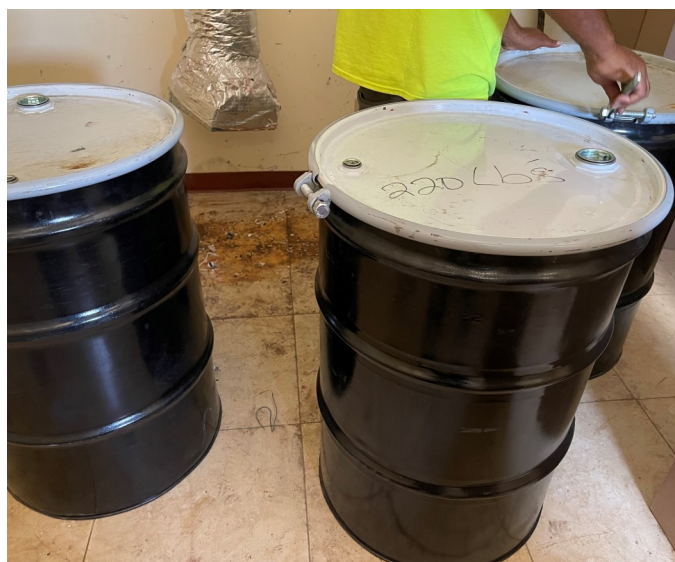
Picture 8 - CHARLES HARDWOOD MEMORIAL COMPLEX, ST. CROIX— At the 2nd Level Main Building Area, there were three (3) 55-gallon black steel drums with lids containing "Ballast" which were removed from aluminum frames.
