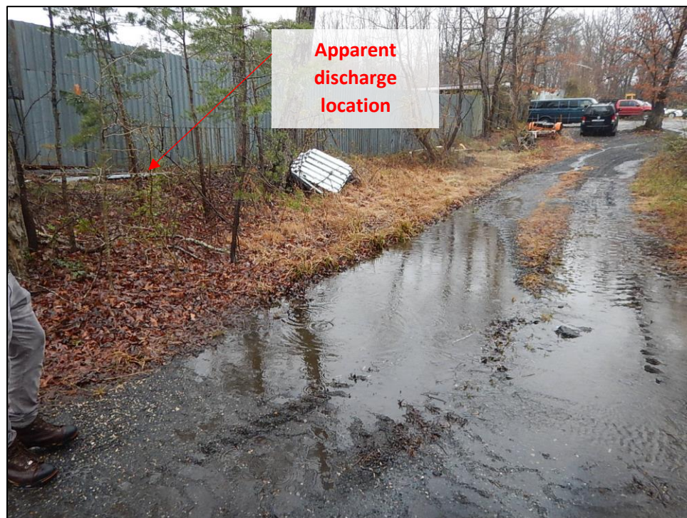
DSCN4113. View, facing northeast, of stormwater pooled outside of the Facility's southeastern perimeter. Note the apparent discharge location. Photograph was taken offsite.
