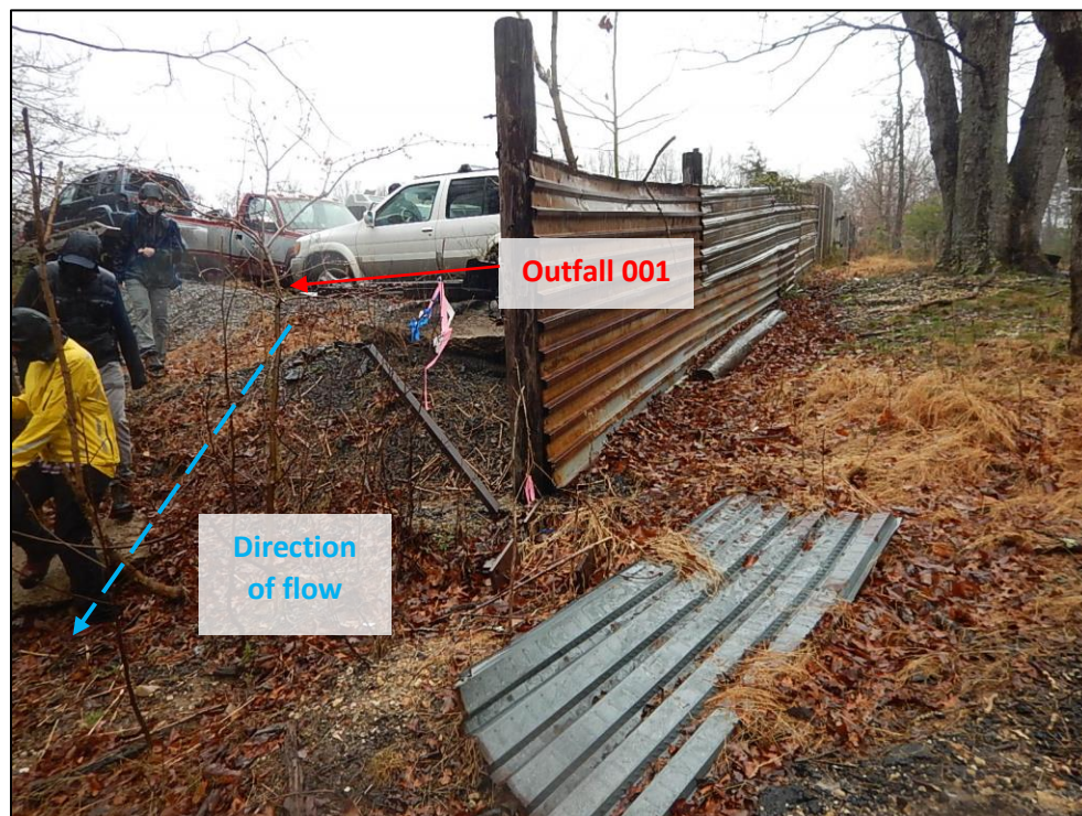
DSCN4094. View, facing northeast, of Outfall 001 (as designated in the previous permit) at the Facility's southern corner. Note the collapsed fence.
