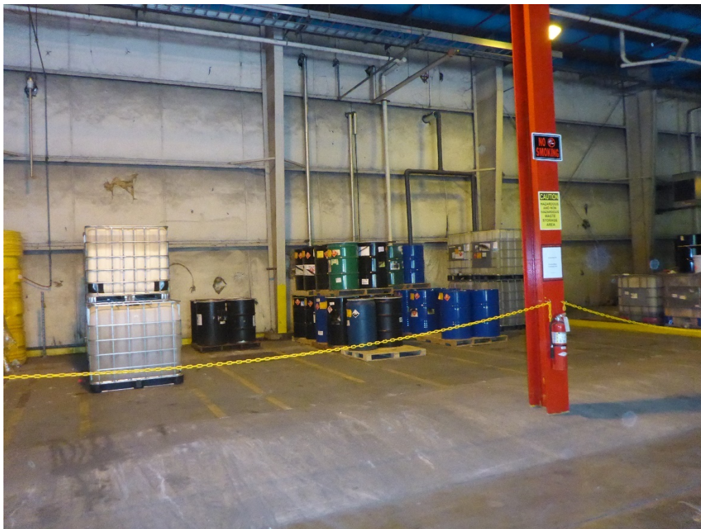
Photo 3: Warehouse CAA on concrete floor surrounded on three sides with a concrete berm and a concrete hump on the fourth side. Yellow lines are painted on the floor to designate six rows for storing waste containers with aisle spacing. The area was identified with signs which read “caution, hazardous and non-hazardous waste storage area,” and “no smoking.”
