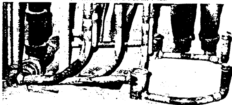
These space-saving lead wastes and vents for back-to-back bathrooms were prefabricated in the plumber's shop located on the site of the Kansas City apartment project, Summit House on the Plaza.
