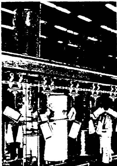
Phosphoric acid pickling line in use in the Peoria, Ill. plant of Caterpillar Tractor Co. Regenerating tank is the tall tower at left.
