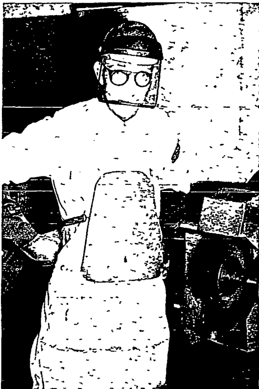
FIG 38-49 — Personal protection for a wire brush operation—the chest plate is made of aluminum
