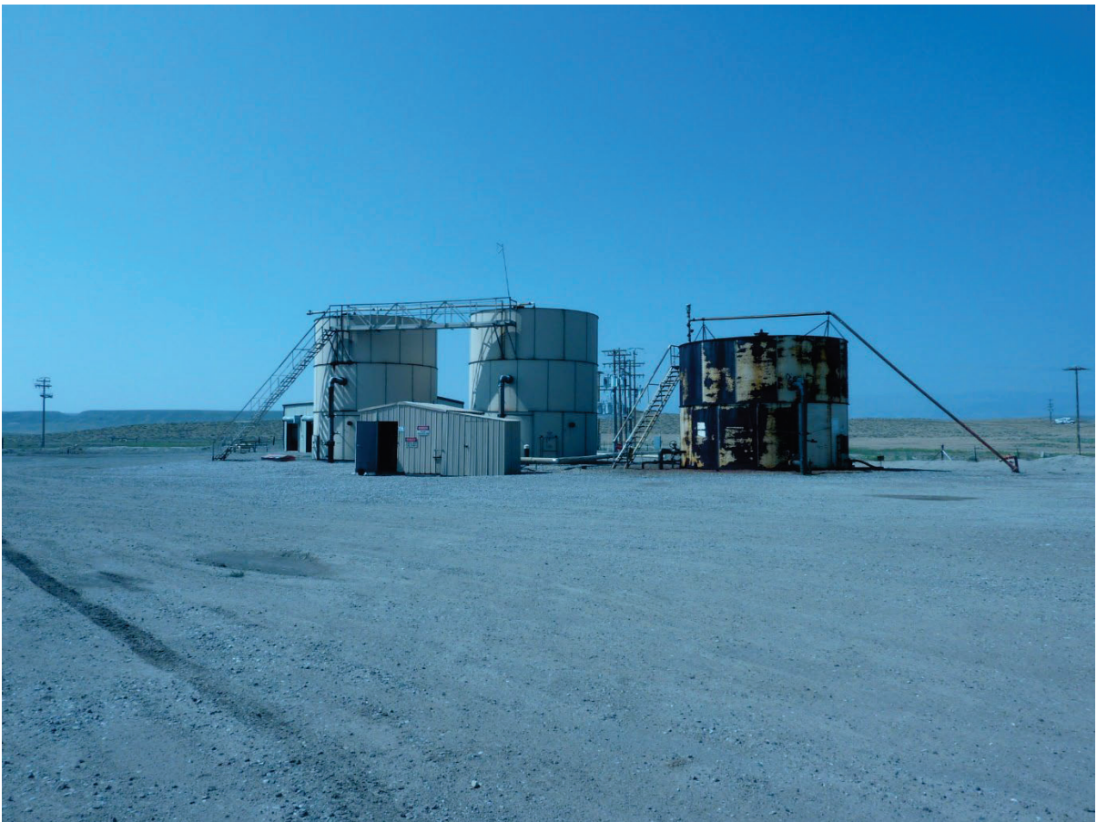
Photo of Water Tanks
