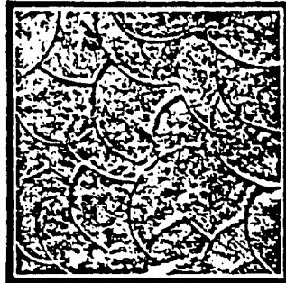
Small Circular Swirls with Toe of Trowel Beginning at Top
