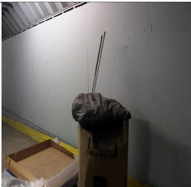
Ramp Area. Inspectors observed two four-foot fluorescent lamps in the container. Photograph 2 taken at 10:06 a.m.
