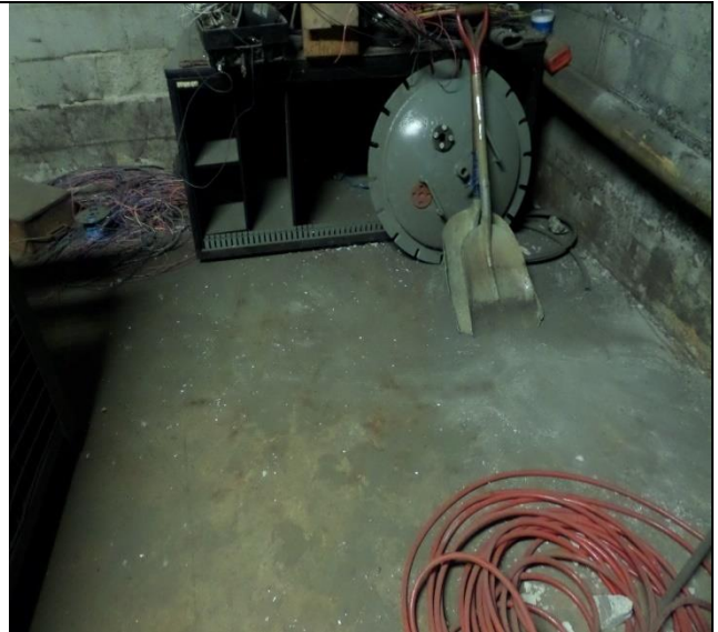
Basement. The inspectors observed Signal cleaned the release of broken lamps to the concrete floor. Photograph 14 taken at 12:07 p.m.
