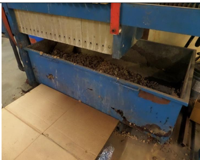
Zinc Wastewater Treatment Line. Inspectors observed zinc solids generated from the filter press were accumulated in a container that was not in good condition. Signal representatives indicated the solids are nonhazardous waste. Photograph 6 taken at 10:57 a.m.
