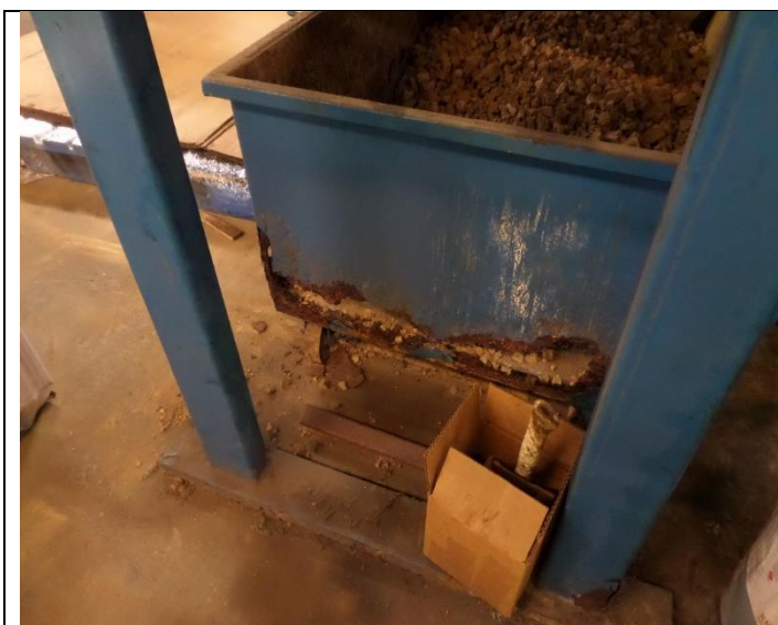
Zinc Wastewater Treatment Line. Inspectors observed zinc solids generated from the filter press were accumulated in a container that was not in good condition. Inspectors observed the release of solids to the floor. Signal representatives indicated the solids are nonhazardous waste. Photograph 7 taken at 10:59 a.m.
