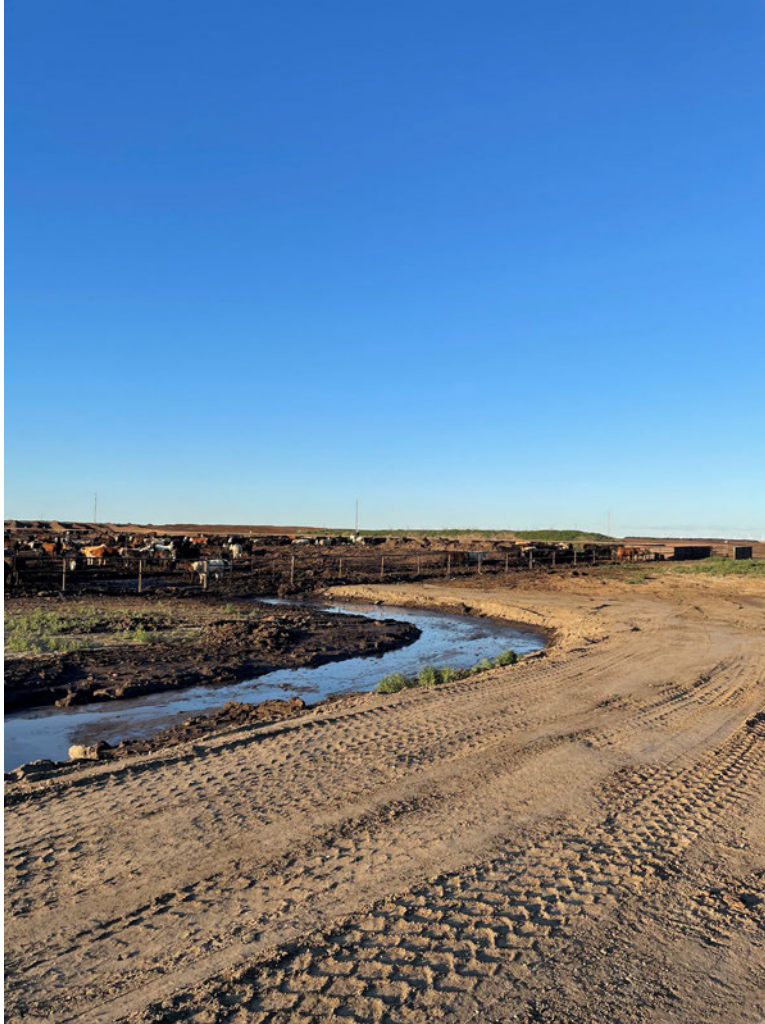
Photo 6. View of settling cell SC-12 after the facility regraded the settling cell.
