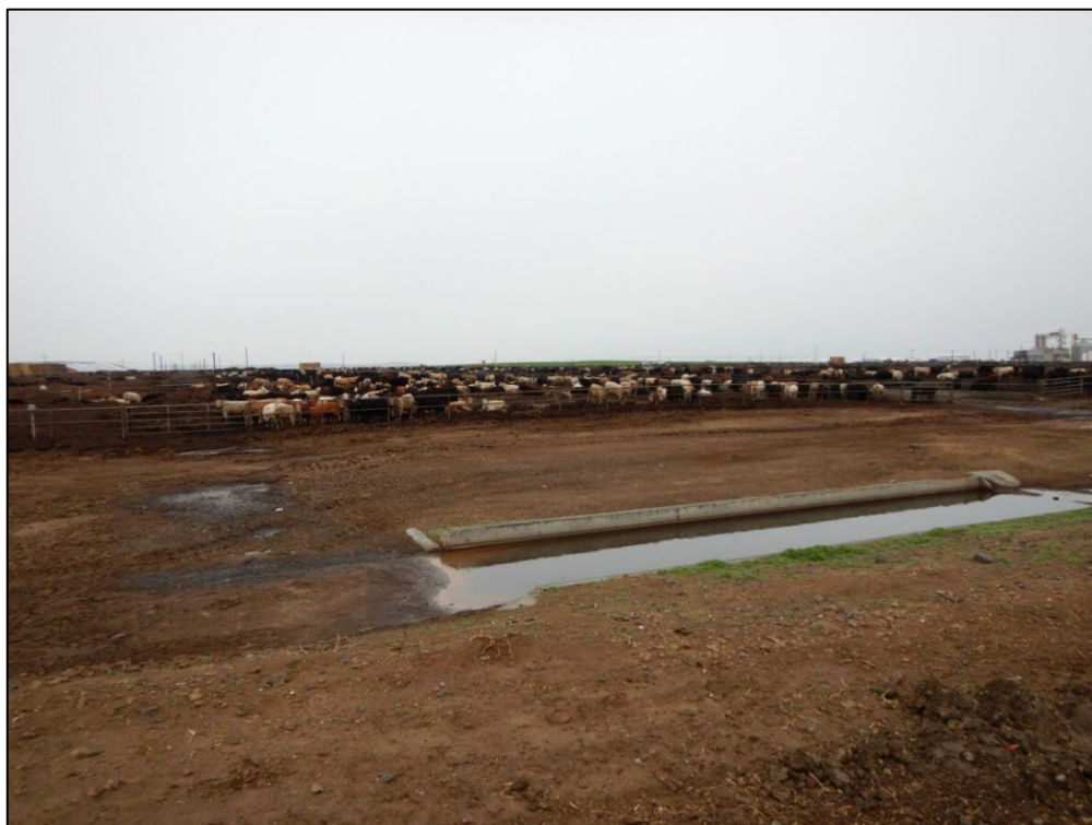
Photograph 25. Settling cell SC-1 receives runoff from the adjacent cattle pens, view looking north.
