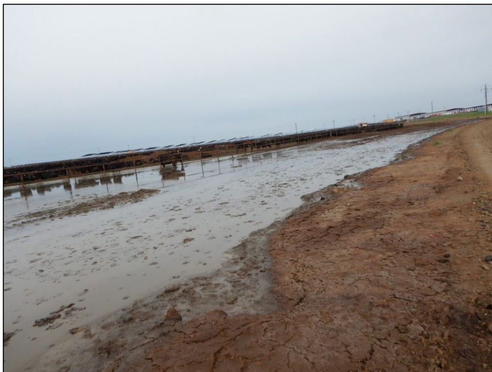
Photograph 3. Alternative view of wastewater within conveyance ditch CD-6, view looking north.
