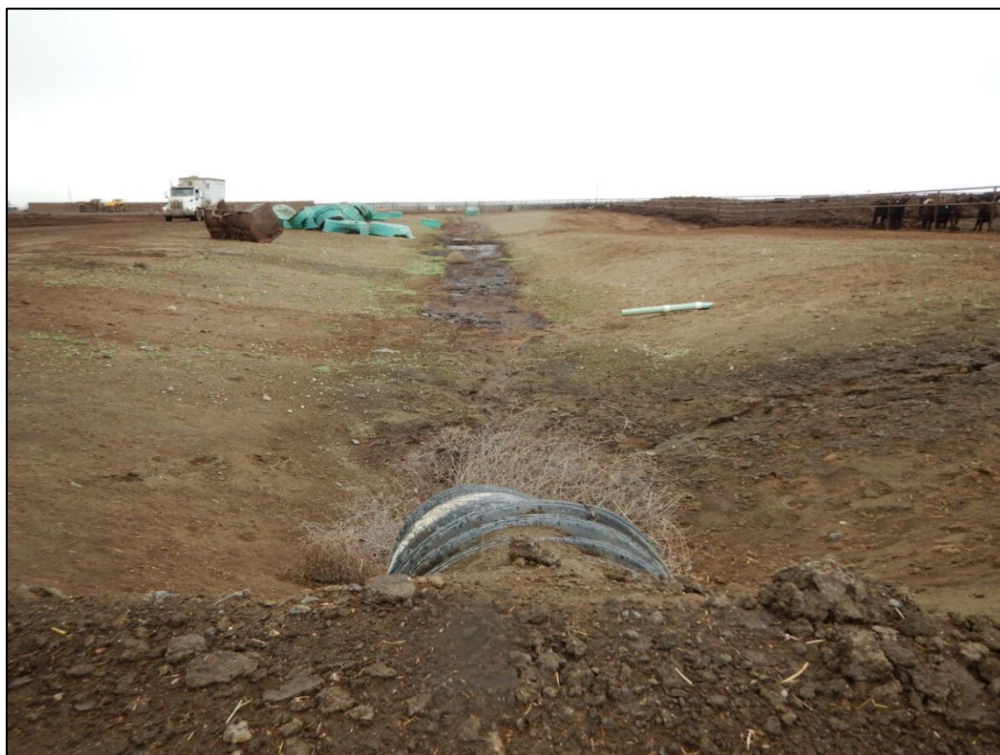
Photograph 13. Conveyance ditch CD-2a conveys cattle pen runoff to settling cell SC-13, view looking east.
