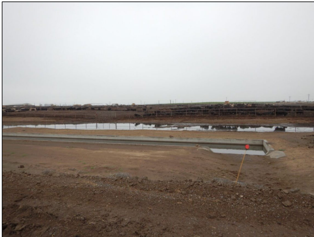
Photograph 21. Settling cell SC-5 and settling cell SC-11 receive runoff from the adjacent cattle pens, view looking north.
