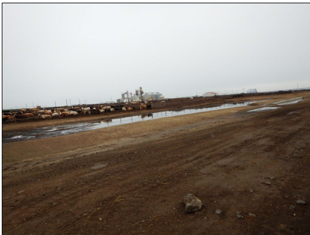
Photograph 22. Settling cell SC-4 and settling cell SC-10 receive runoff from the adjacent cattle pens, view looking northeast.
