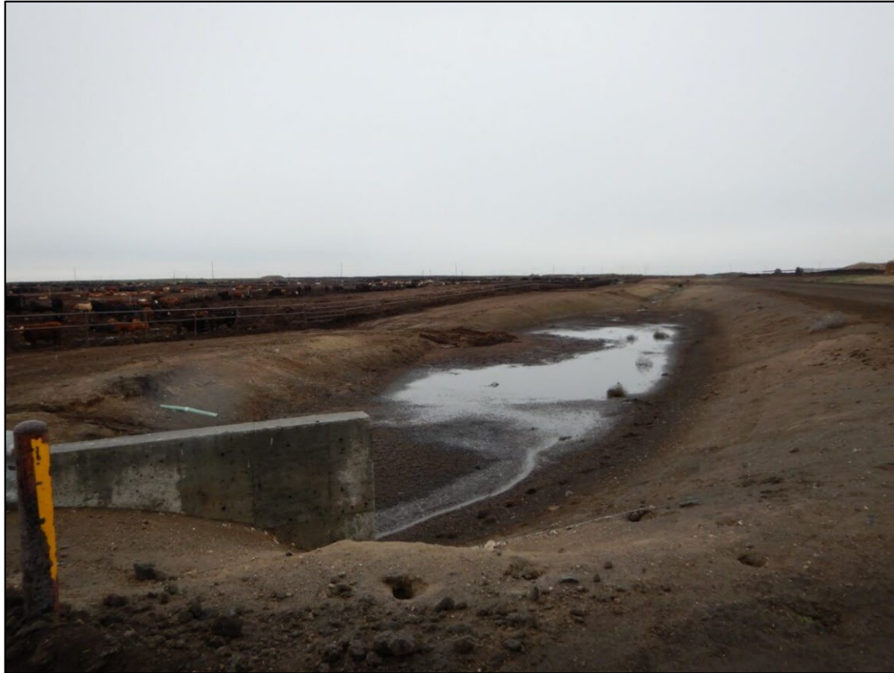
Photograph 17. Alternative view of settling cell SC-14, looking west.
