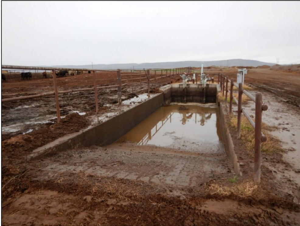
Photograph 33. View looking north at the Pasture Pond collection pit which receives runoff from the adjacent cattle pens. Wastewater is pumped from the collection pit to the Pasture Pond.
