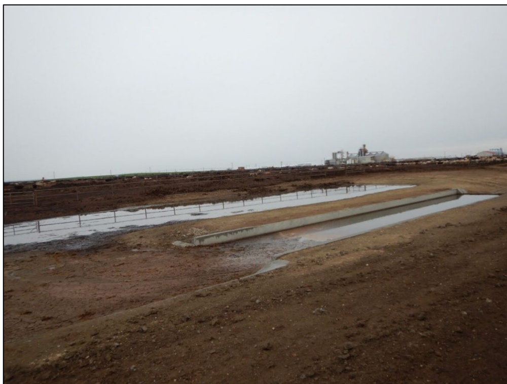
Photograph 24. Settling cell SC-2 and settling cell SC-9 receive runoff from the adjacent cattle pens, view looking northeast.
