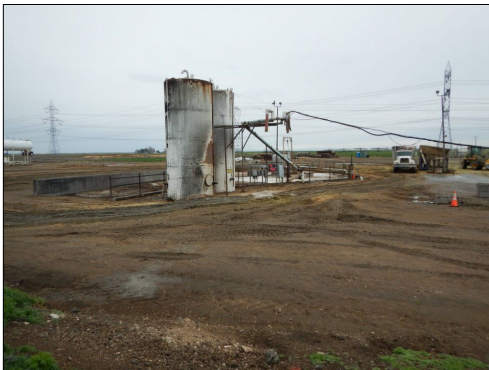
Photograph 36. View looking south at the potato slurry tank at the facility's pasture production area. Potato processing waste is hauled to the facility and stored in this tank for feeding the cattle. Spills or overflows from this tank would flow to the Collection Pit.
