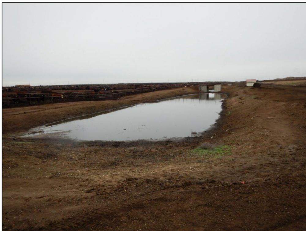
Photograph 19. Settling cell SC-16 receives runoff from the adjacent cattle pens, view looking west.
