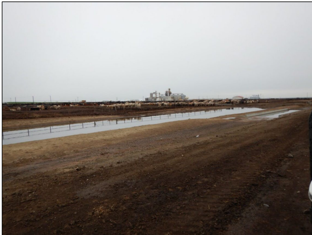
Photograph 23. Settling cell SC-3 and settling cell SC-9 receive runoff from the adjacent cattle pens, view looking northeast.
