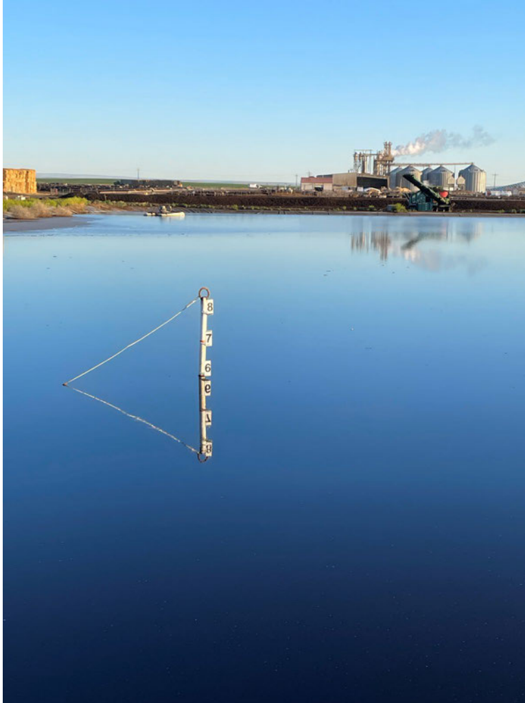
Photo 5. The depth marker in Lagoon 1 with a mark identifying the freeboard level at 7.0 feet. The pumping level mark is below the surface of the wastewater.
