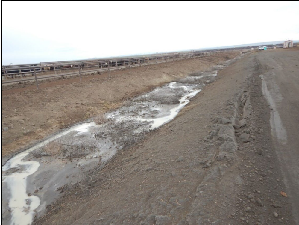
Photograph 29. Alternative view of conveyance ditch CD-3, immediately downstream of Photograph 28, view looking south.
