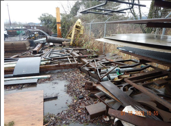
Photo #: 15 (DSC0541) Description: Facing northwest, overview photo of the outside of the Facility, largely used as storage with a mixture of scrap metal and debris on the ground.
