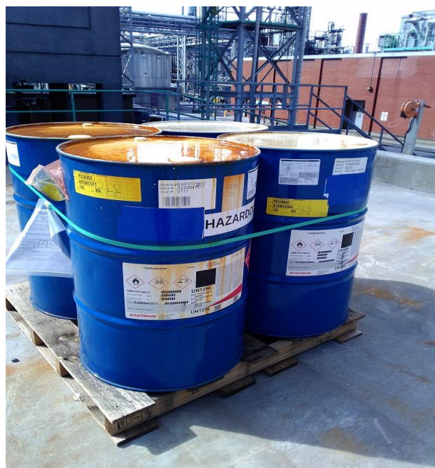
Photo 5: Building 244 – four drums of waste triethylamine labeled as “Hazardous Waste”
