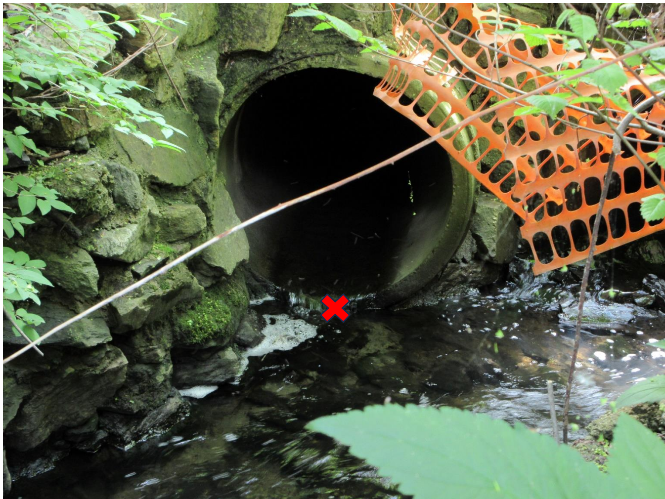
Photo 6: LQ-06BL (photo taken 05/28/2024 at approx. 13:48) Outfall located near 10 Crane Street, discharging into an unnamed stream that discharges into Lake Quinsigamond. Sample points are indicated by a red X.
