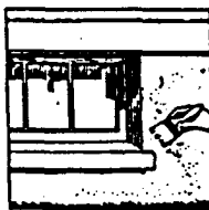
To protect concrete surfaces
