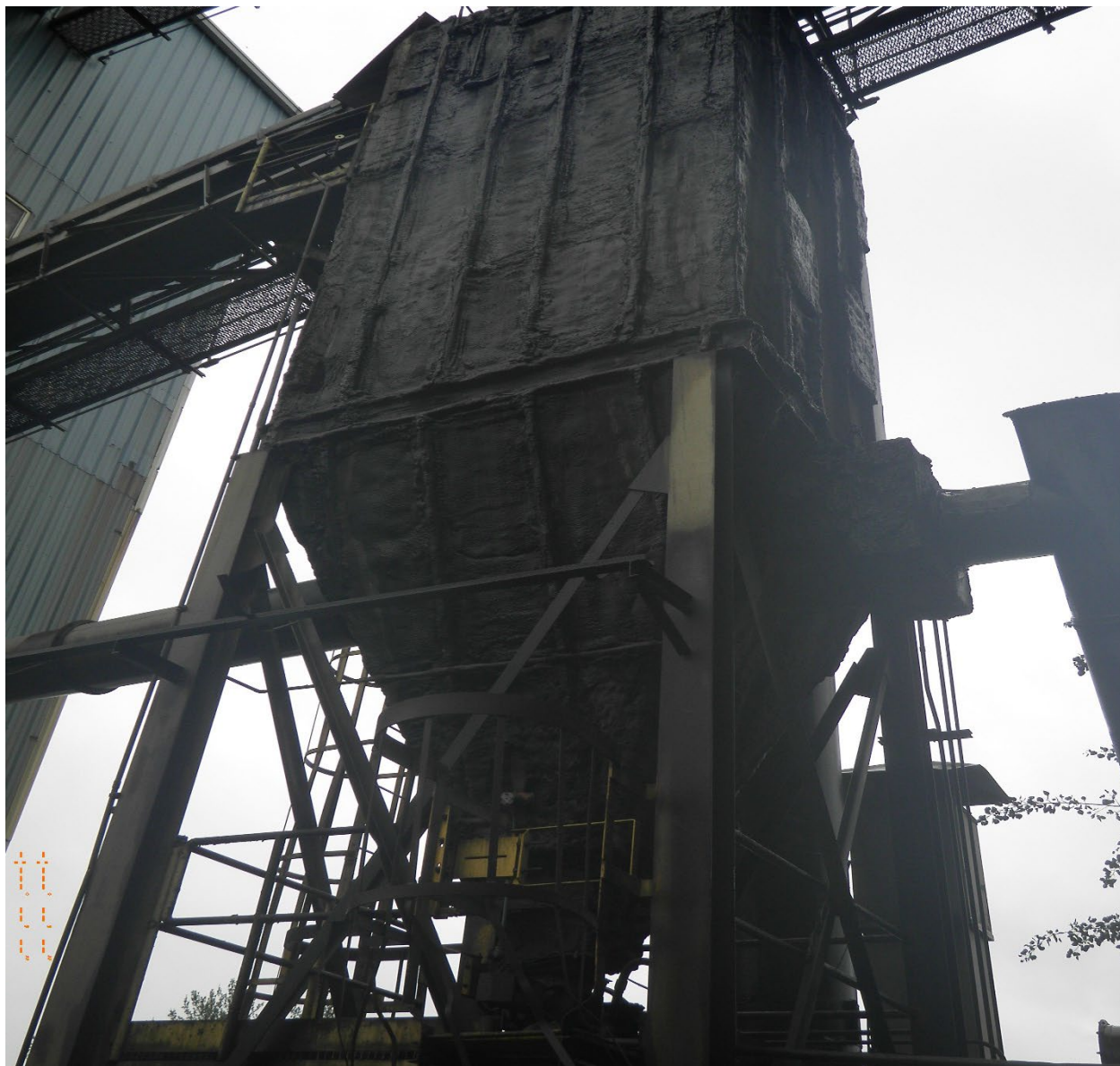
5. Hopper outside of Crusher Building – Scrubgrass Generating – 6/7/22
