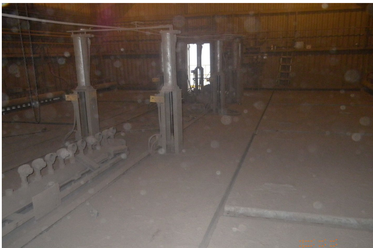
21. Top of Boiler 1 Baghouse –Scrubbygrass Generating – 6/7/22
