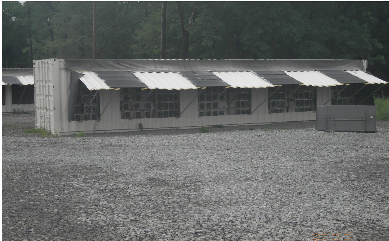
23. Data Center Storage Container with Computers – Scrubgrass Generating – 6/7/22
