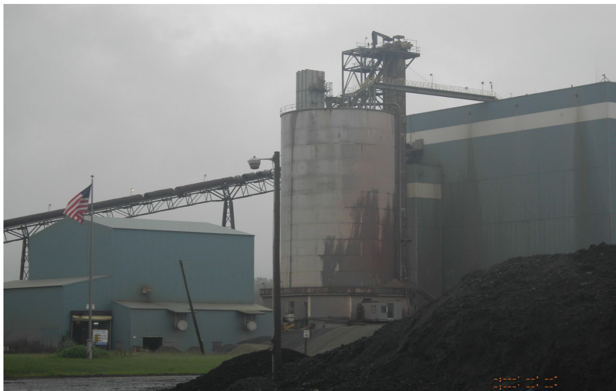
4. Ash Silo – Scrubgrass Generating – 6/7/22
