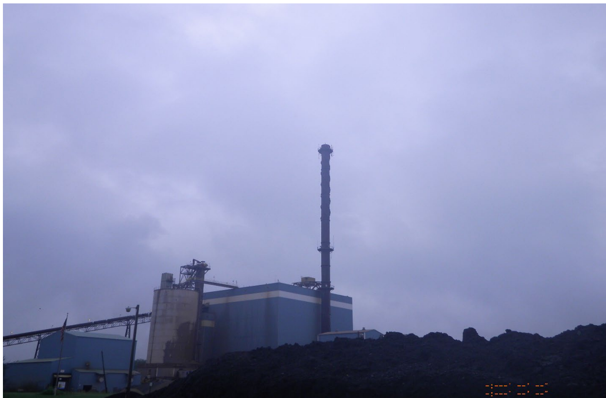
3. Boiler 1 & 2 Combined Stack – Scrubgrass Generating – 6/7/22
