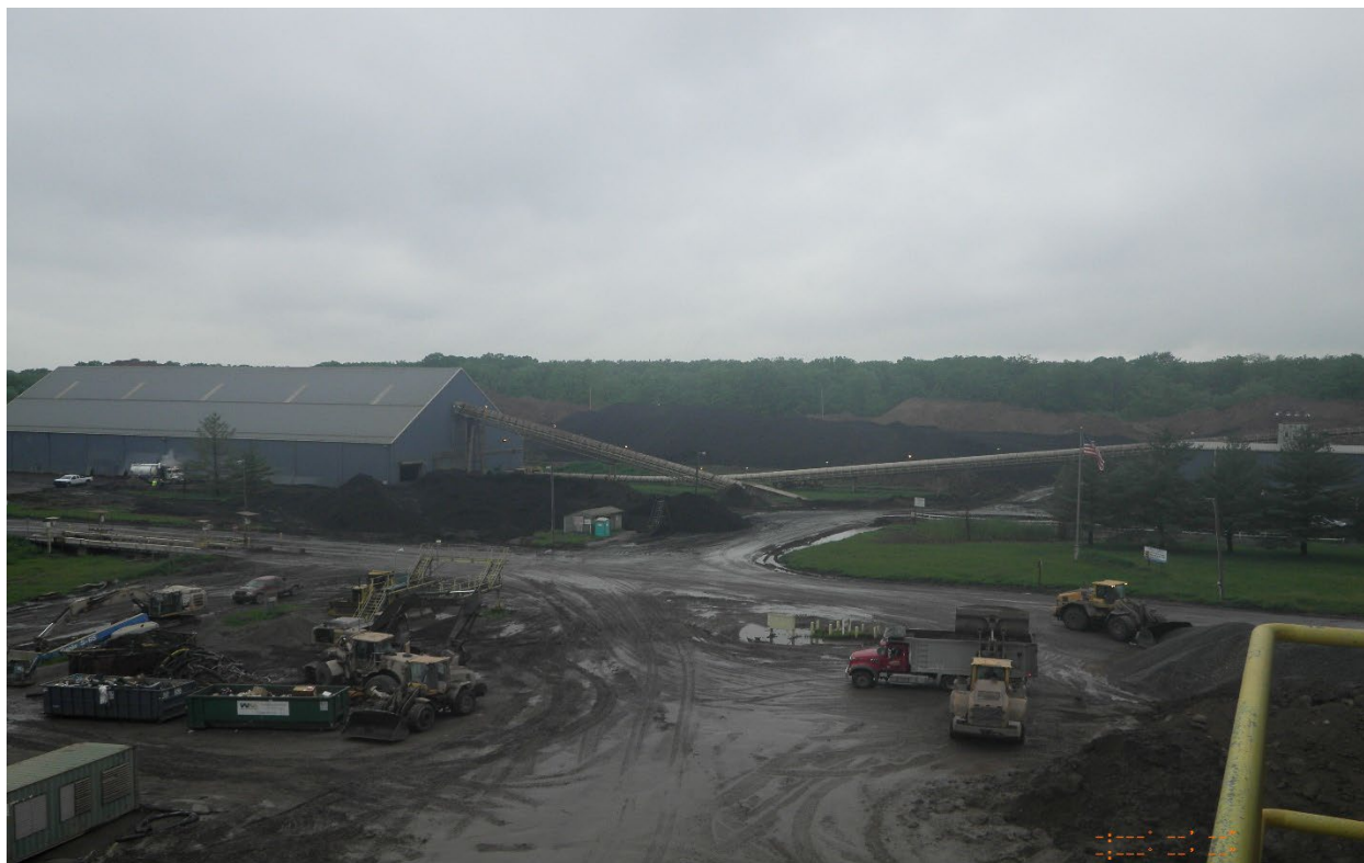
22. Coal Storage Building & Coal Pile – Scrubgrass Generating – 6/7/22
