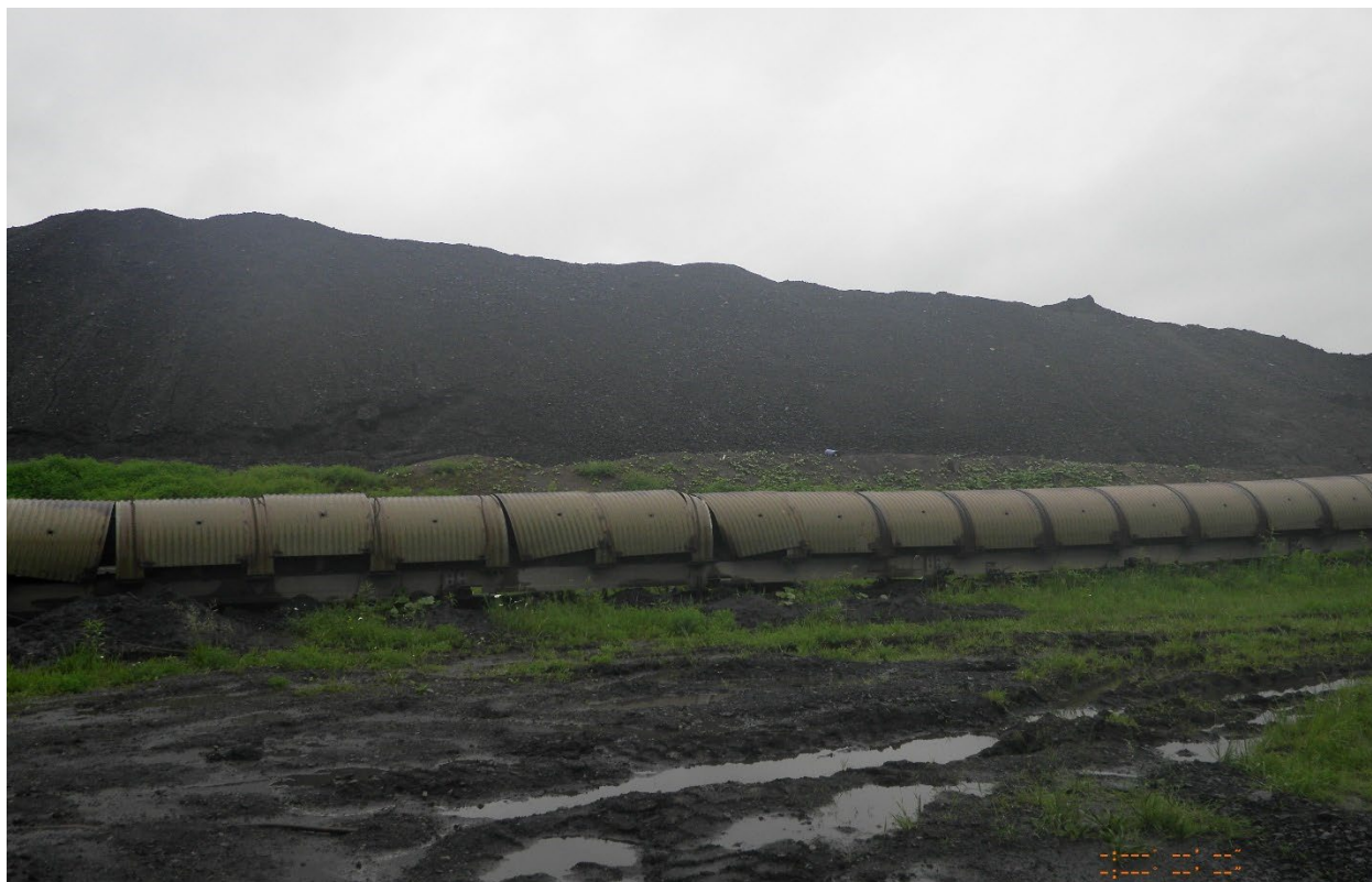
1. Waste Coal Pile & Covered Conveyor – Scrubgrass Generating – 6/7/22
