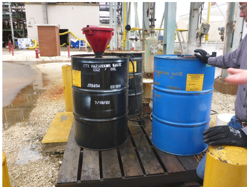
Photo 7: Two SAAs in the Crystex Plant Area. One SAA is used to accumulate hazardous waste liquids that are generated from decontamination and maintenance activities as D001, D018 hazardous waste flammable liquid (oils, xylene), the other is used to accumulate used filters that are generated in the Crystex Plant as D001, D018 hazardous waste solids.
