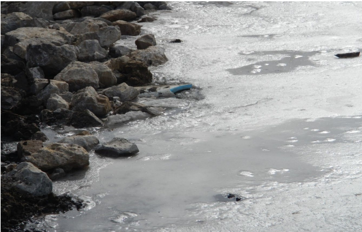
DSCN1071, Inlet of 12-inch pipe beneath Stream Crossing SC #3
