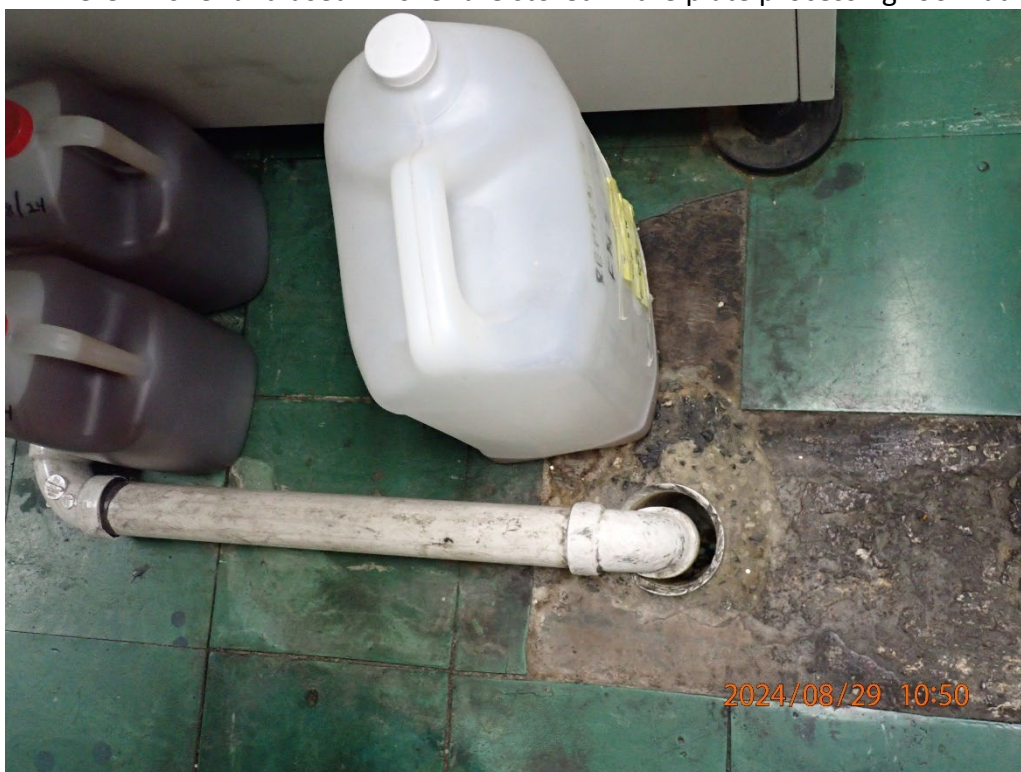
Photograph 5: Process waste pipe entering system at RR Donnelley.
