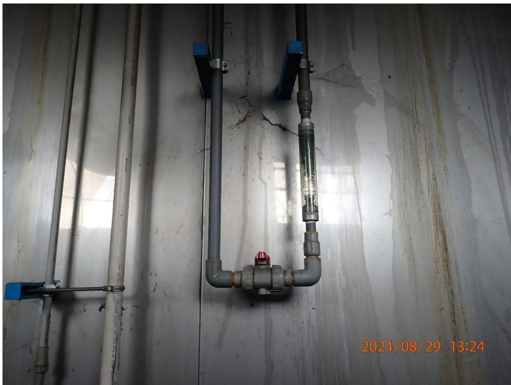
Photograph 14: Levers that control water levels on powder coat lines at Lepko.
