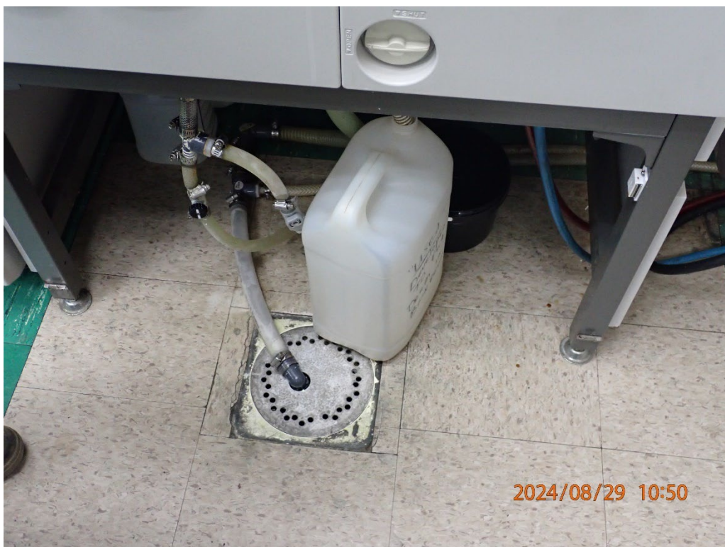
Photograph 6: Process waste entering drain at RR Donnelley.
