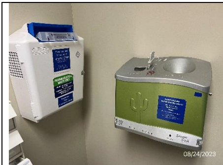
Figure 1: 10:00 AM Medication Room One 1-gallon container with hazardous waste label and indication of the hazards of the contents observed.
