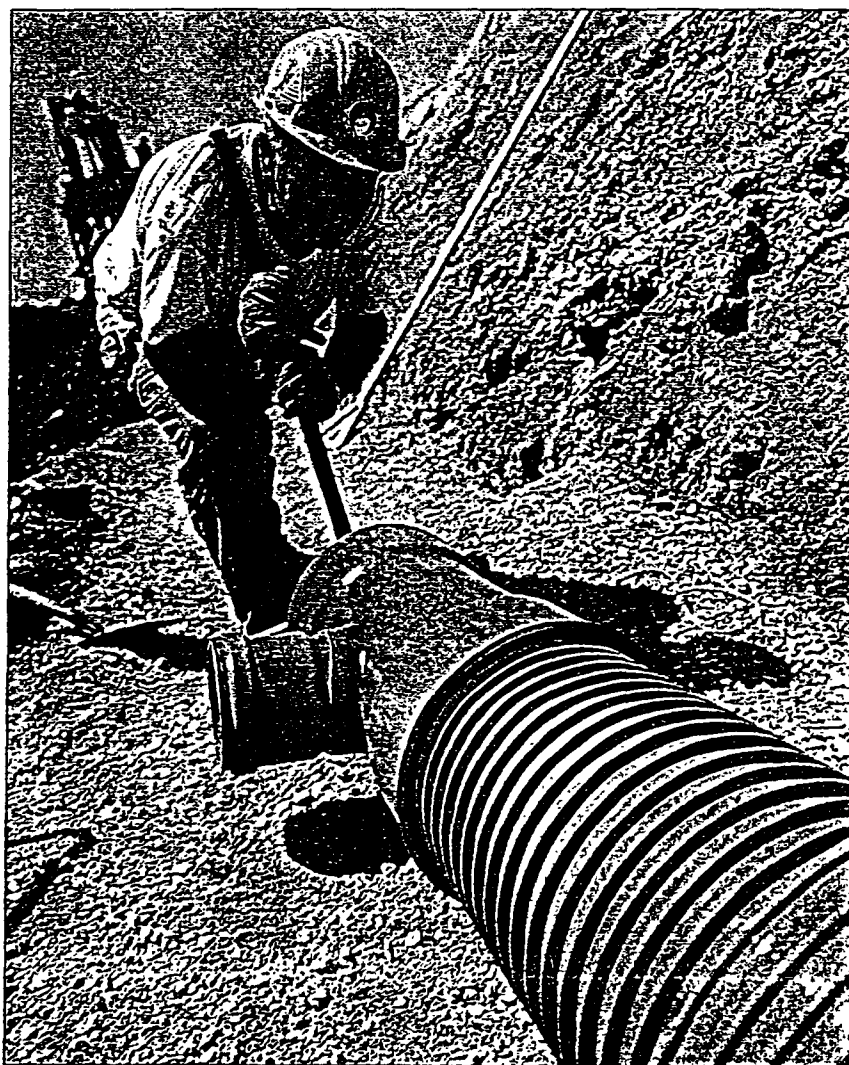
An unidentified worker installs a PVC Ultra-Rib sewer pipe with a PVC fitting. This type of PVC pipe complies with ASTM Standard F794.
