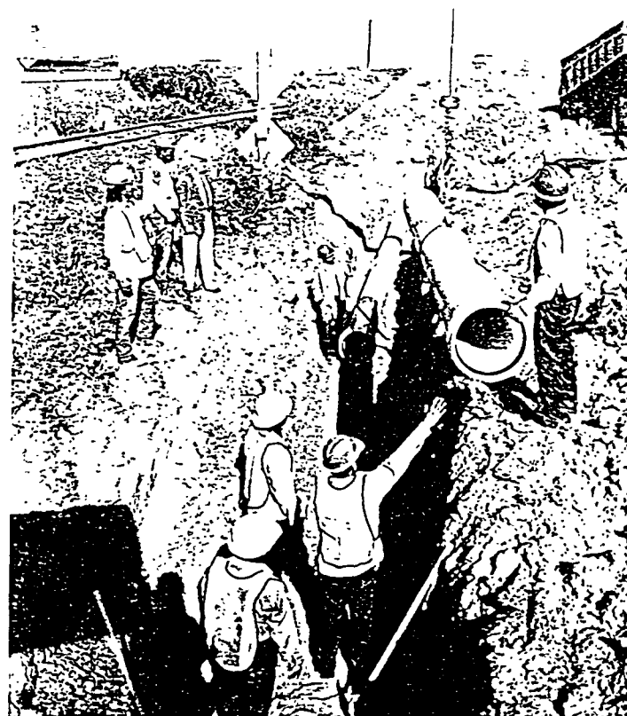
An ocean-going freighter passes through the Avery Point Channel to the Port of Corpus Christi (left), as Paul Werner supervises PVC pipe installation. By replacing 8-inch cast iron pipe with 16-inch vinyl pipe twice its diameter, Werner was able to double the flow of water in two lines joining the Point to the city's main water system.
