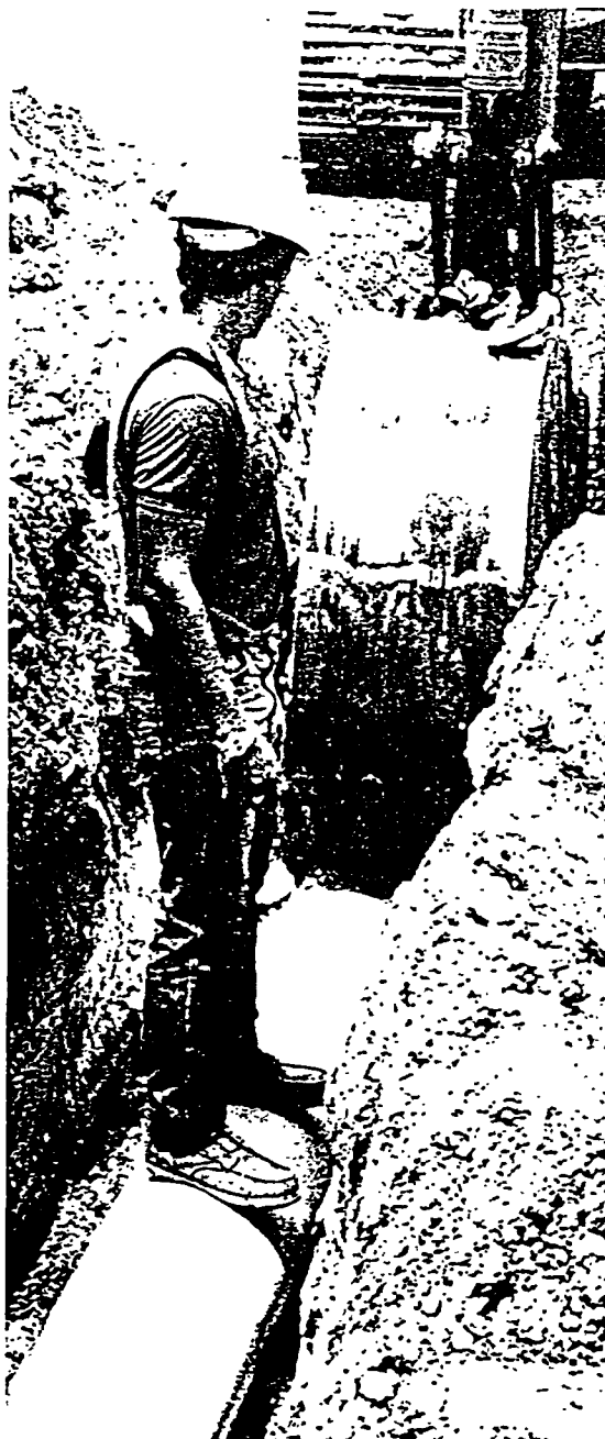
A joint of 12-inch PVC (vinyl) pipe is prepared for installation in a $28 million expansion project that will double the size of Cape Coral, Florida's water system.
