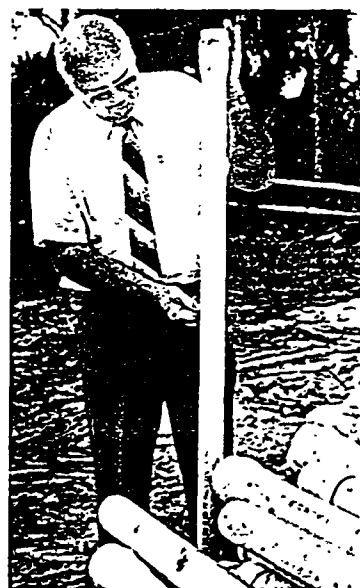
Twelve-inch PVC pipe was specified to replace clay pipe in an Ormond Beach, Fla., gravity sanitary sewer system. Jack Dillard (left) supervises installation.
