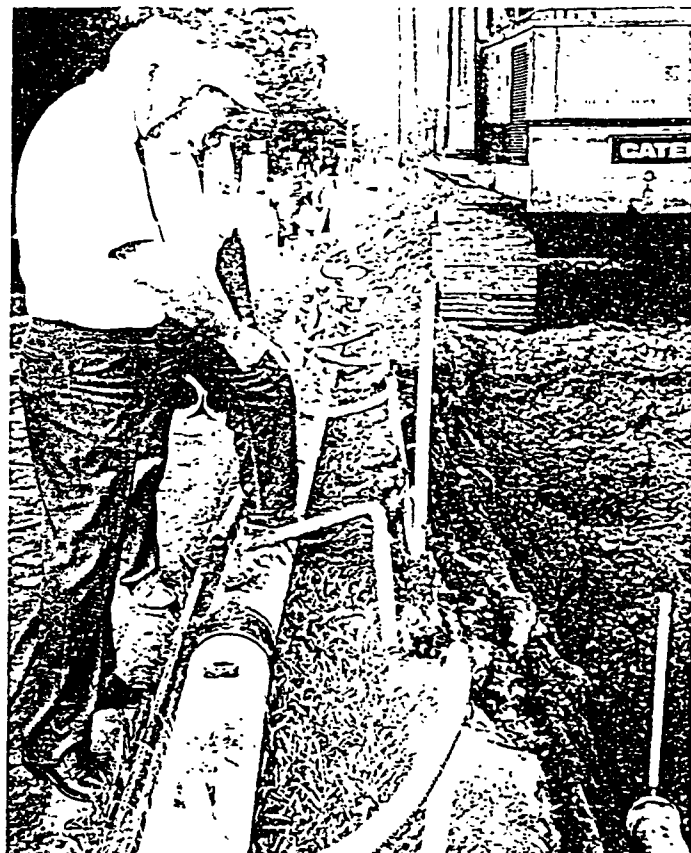
Twelve-inch PVC pipe was specified to replace clay pipe in an Ormond Beach, Fla., gravity sanitary sewer system. Jack Dillard (left) supervises installation.
