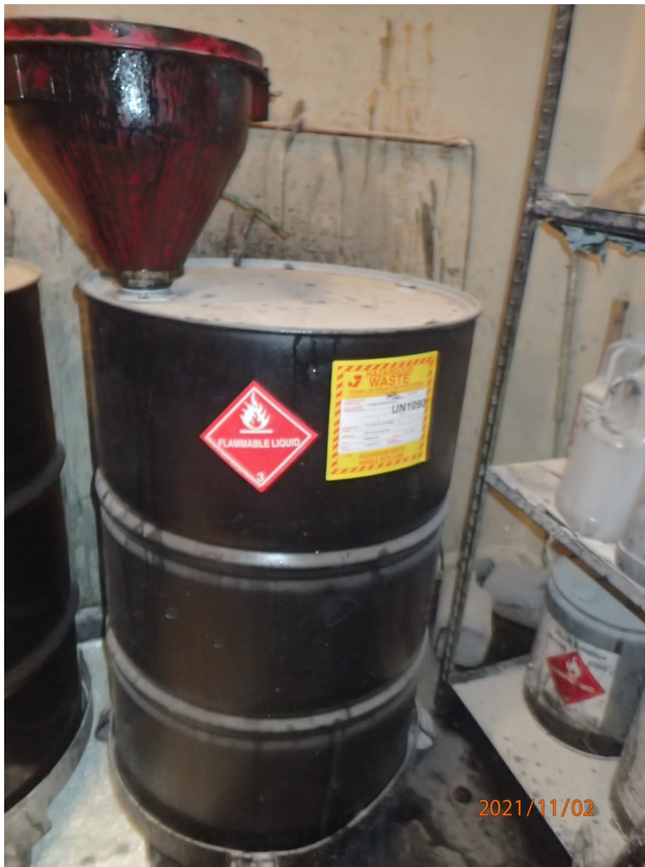
Photo 3: One (1) 55-gallon SAA hazardous waste drum containing waste acetone. The container was closed and labeled with the words "Hazardous Waste" and marked with an indication of hazard.
