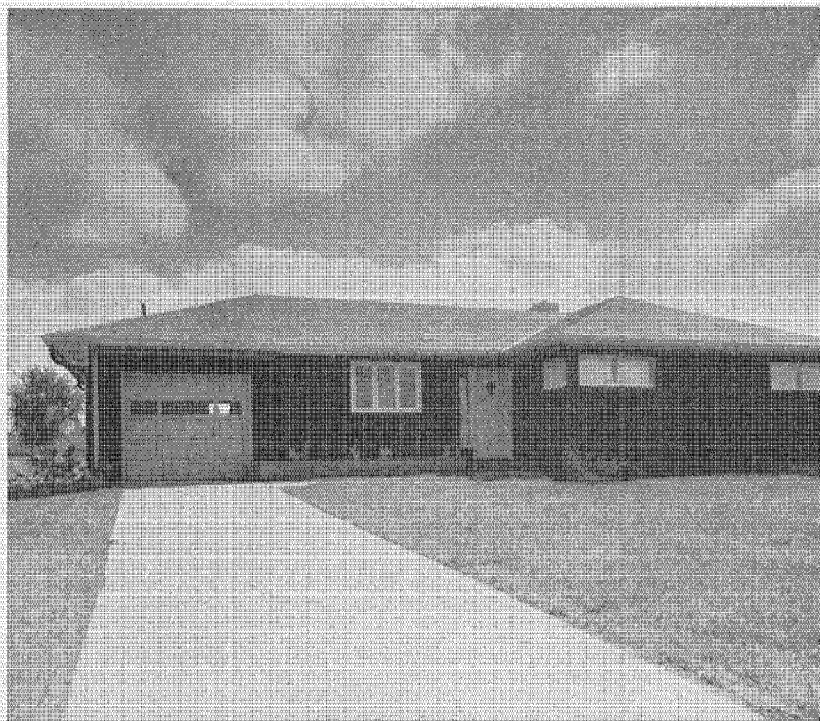
Here's the completed house, one of 500. Projects like this illustrate trend to air conditioning in medium-price field.
