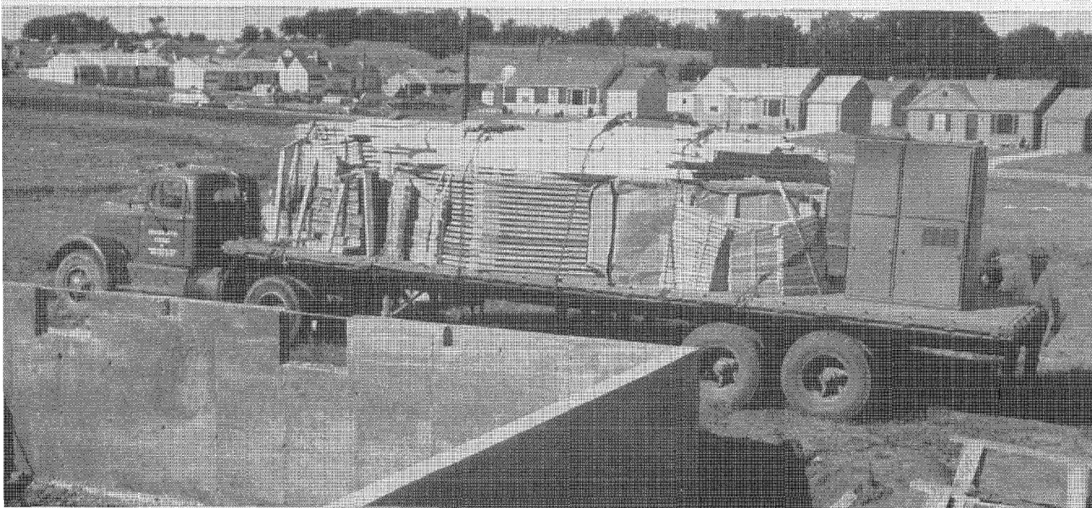
Shell of house, complete with central air-conditioning unit, arrives by truck at a Kansas development. In 1952, 10,000 air-conditioned homes were built in the U.S. Outlook for '53: several times that many.
