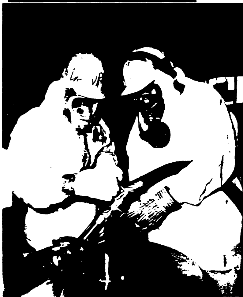
Fernald workers hook up lines to a vacuum to remove hold-up material from equipment in Plant 4 - the next building slated for demolition.
