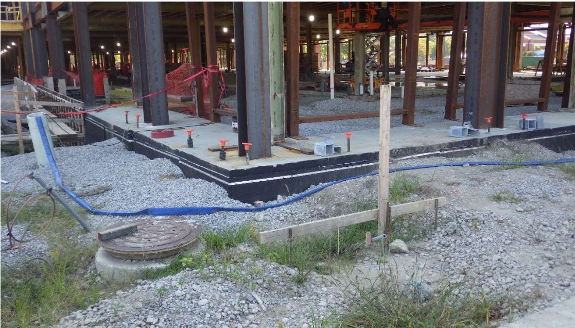
24: RIMG0024 Description: Blue hose from white vertical pipe (left) to ajar manhole (right). Location: West side of building 1600 construction site. Camera Direction: Northeast Date/Time: 09/18/2024 10:14 AM
