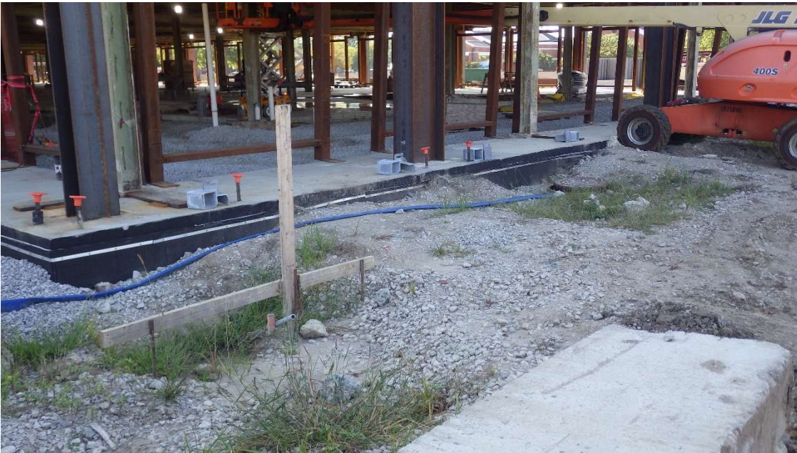
25: RIMG0025 Description: Blue hose from white vertical pipe (left) to ajar manhole (right). Location: West side of building 1600 construction site. Camera Direction: Northeast Date/Time: 09/18/2024 10:14 AM
