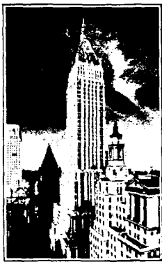
The Bank of Manhattan Building, Wall St., New York
