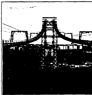
One of the huge 600-foot towers of the Hudson River Bridge, painted with red lead
