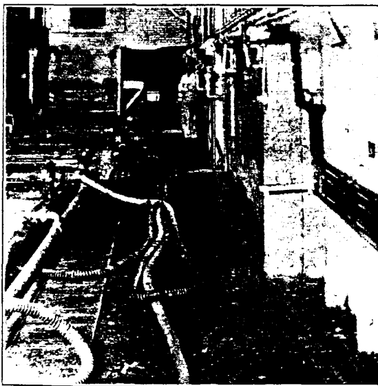
Sheet lead flooring in a white lead plant at East Chicago, Indiana
