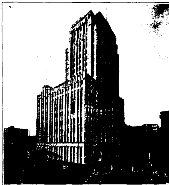
The Washington Athletic Club, Seattle, just completed, is painted throughout with white lead and oil
