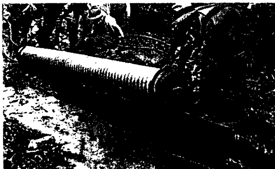
Installing pipe line in conduit under railroad.
