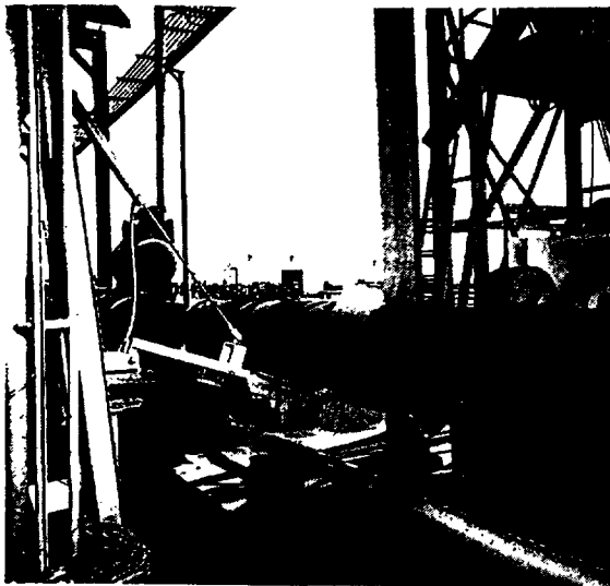
Cement-mortar coating being added to steel pipe.
