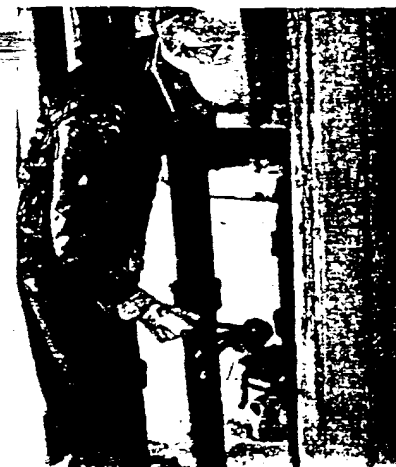
The plumber is connecting the lead sink waste to the stack. Note the two space-saving 90 deg. offsets in the lead pipe.
