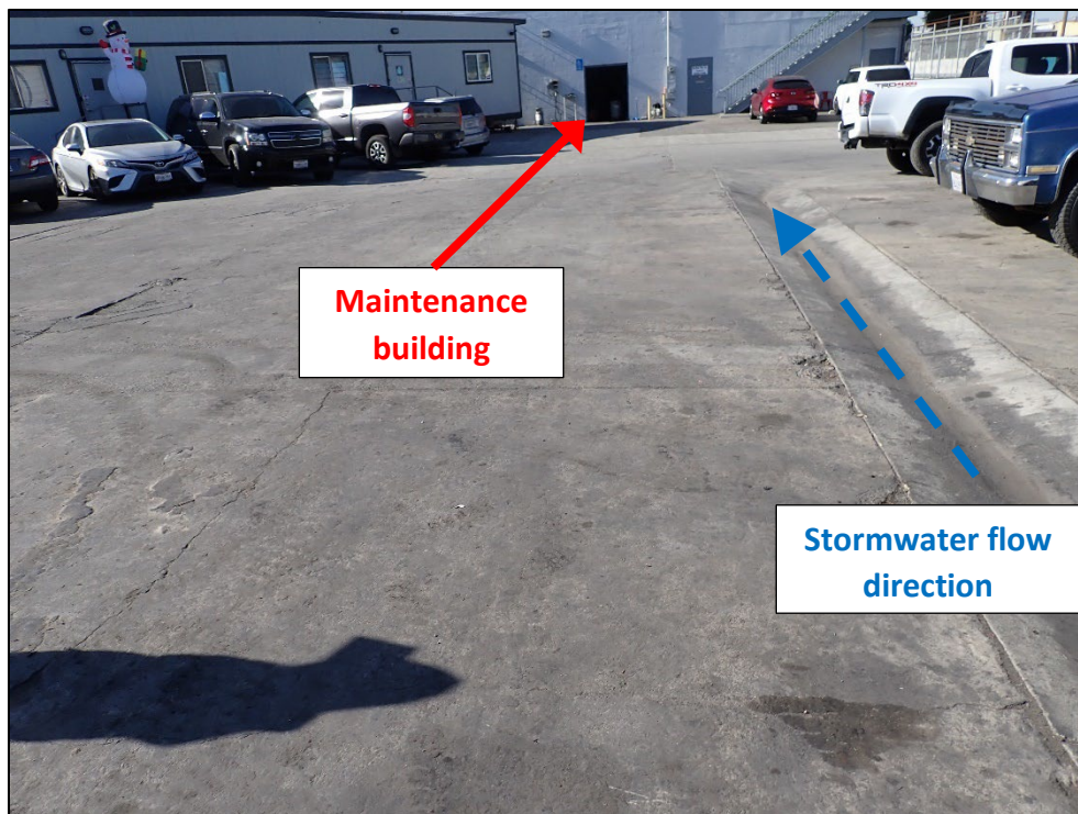
Photograph 12. View, facing west, of the center of the Facility. This area had a shallow trench that conveyed stormwater towards the entrance/exit of the Facility.
