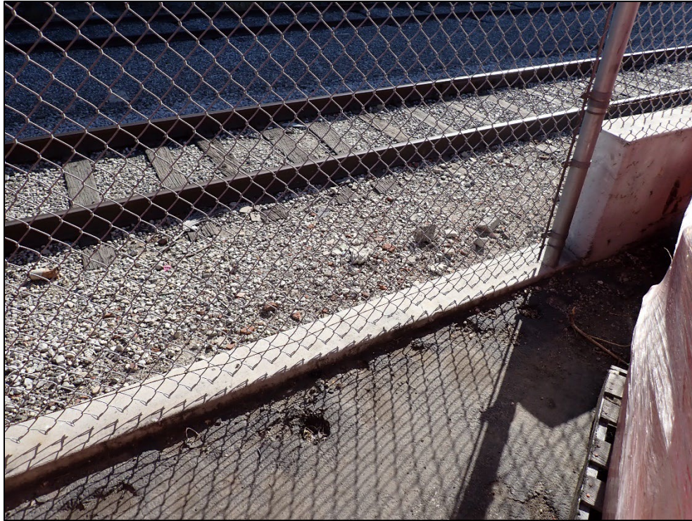
Photograph 5. View, facing south, of the Facility's southern boundary. The perimeter of the Facility, aside from the entrance/exit, was enclosed by a concrete wall or concrete berm.
