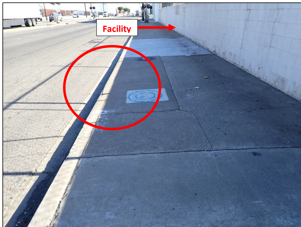
Photograph 14. View, facing east, of a curb inlet located directly to the east of the Facility's entrance/exit. The curb inlet connects to the Los Angeles County MS4.
