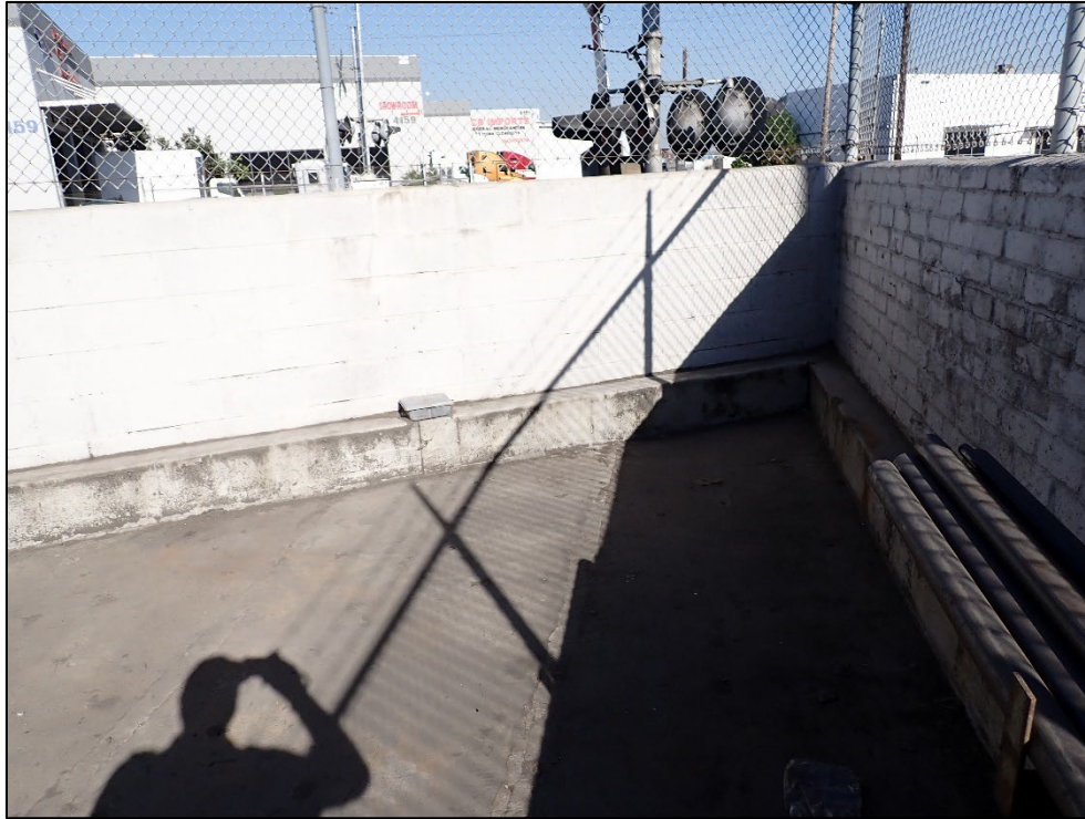
Photograph 11. View, facing north, of the Facility's northeastern boundary.
