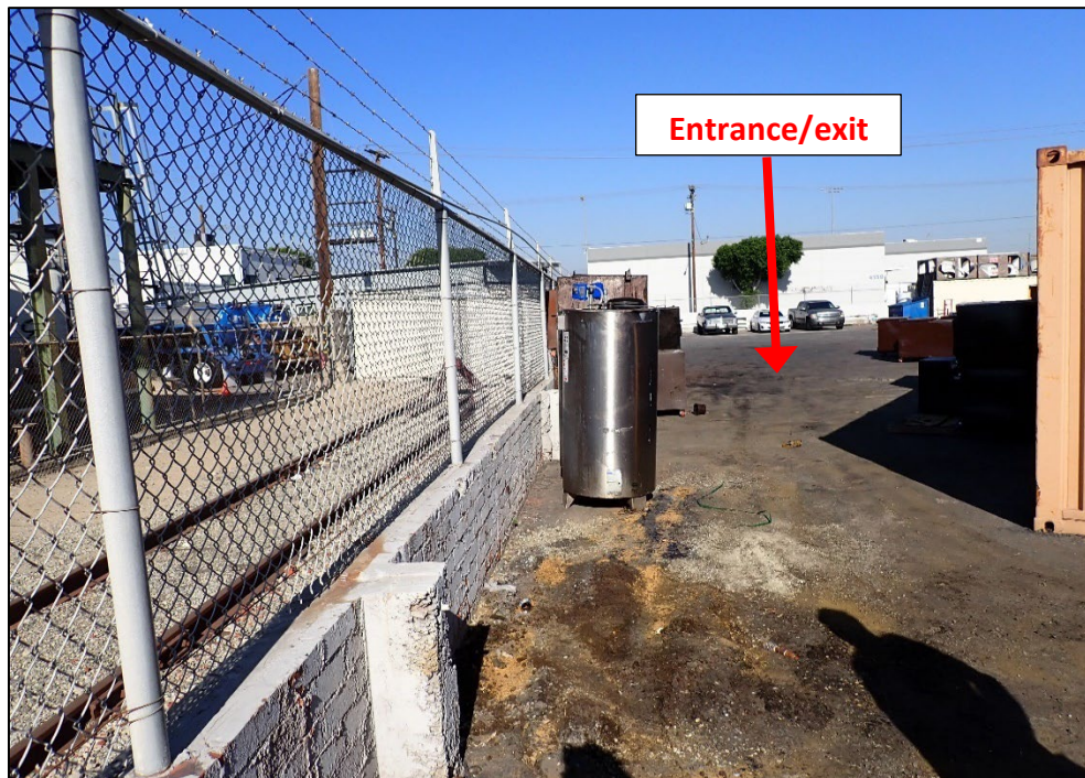
Photograph 6. View, facing north, of the Facility's western boundary. Note the spilled used cooking oil on the ground surface adjacent to the 100-gallon used oil tank.
