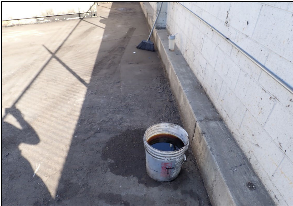
Photograph 10. View, facing north, of a 5-gallon bucket containing used cooking oil stored without cover and exposed to stormwater. Note the staining on the ground around the bucket.
