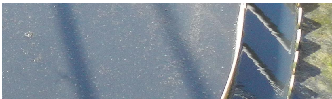
Figure 8. Top bottom photos show gray coloration and clumps of solids (sludge) floating at the surface.
