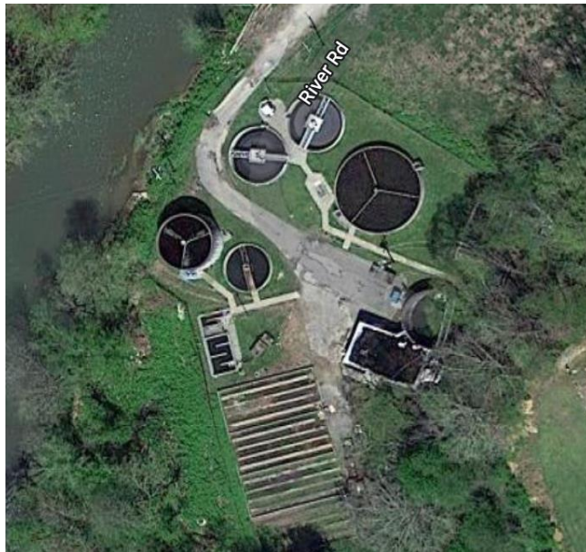
Figure 1: Aerial Display of the WWTP
