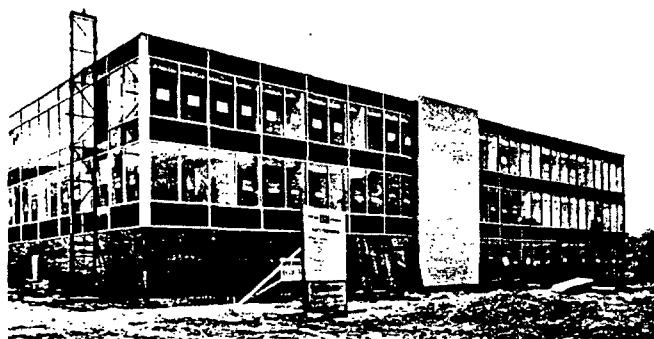
FOUR-STORY REGIONAL HEADQUARTERS of IBM is located on Cincinnati's Victory Parkway, north of central business section. More than 60,000 sq. ft. of SHEETROCK Firecode wallboard was used for interior partitions and facings of exterior walls.
