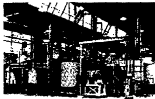
1941 . . . ADDITIONAL CHEMICAL PRODUCTS BUILDING (No. 659) erected to produce many items for military purposes, synthetic rubber and lubricating oils—also providing new processes for some of the intermediates used in color making.
