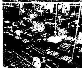
1941 . . . NEW WAREHOUSE (building 28) floor space 215,000 square feet—5 acres erected to provide for stock of many new products being made at Chicago. Modern equipment. Increase in business already crowds this large area.
