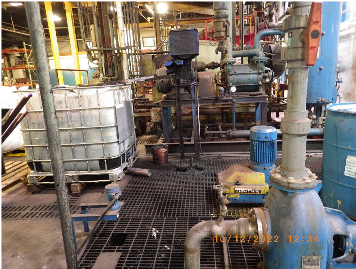
1: APOL0310 Description: East flush pit Location: Building 1, northwest side Camera Direction: Northeast Date/Time: 10/12/22, 12:34 p.m.
