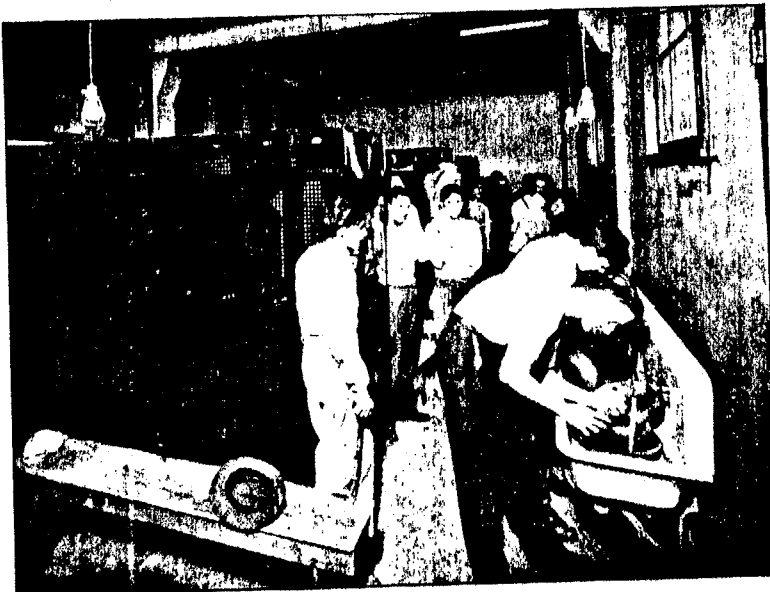
WASHROOM FOR WHITE WORKMEN, ST. LOUIS.
