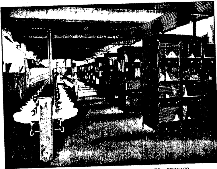
LOCKER AND WASHROOM, SOUTHERN WORKS, CHICAGO.
