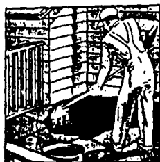
A waterproof coat of Liquid Roof Coating, applied with a 3-knot roof brush, will pay for itself many times over by preventing costly roof repairs.
