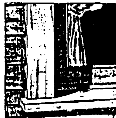
In painting homes it is very important that the paint be properly applied in the areas around windows.
