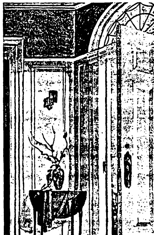
When entrance doors are left open, walls of hallways naturally become covered with an accumulation of dust. This explains the need for painted walls that are washable.
