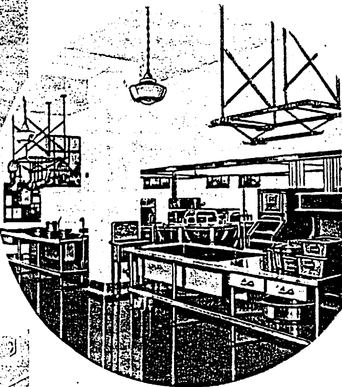
● Kitchen Above: Ceiling—Speed-Wall Semi-Gloss Caen Stone. Walls—Speed-Wall Semi-Gloss Buff. Floor—Florenamel Warm Gray.
