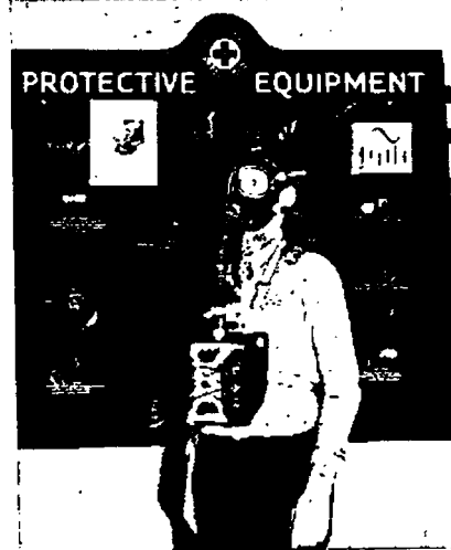
An all-service gas mask may be used in atmospheres where there is no oxygen deficiency.
