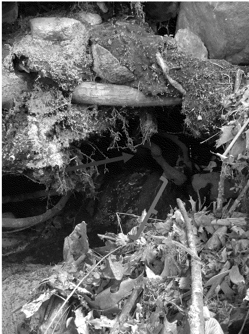
BrookSt (photo taken 5/24 at 11:09 AM): Outfall located at the corner of Brook Street and Queen Avenue flowing into an unnamed stream flowing from Searles Pond. No sample was collected at this location. Outfall is located under the bank on the right side of the photograph (indicated by a red arrow). Discharge flow is visible and is indicated by a blue bracket.
