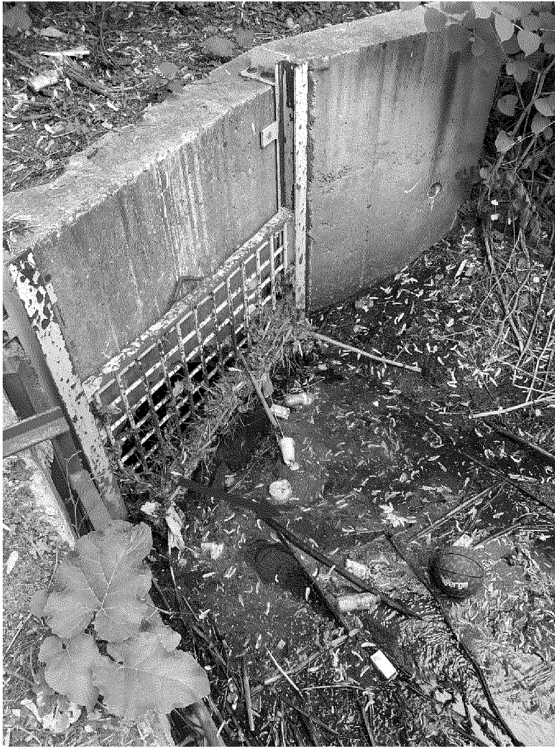
76Swan (photo taken 5/24 at 11:21 AM): View of gated culvert opening where the stream coming from Searles Pond begins to flow underneath the parking lot. Sample point is indicated by a red arrow.
