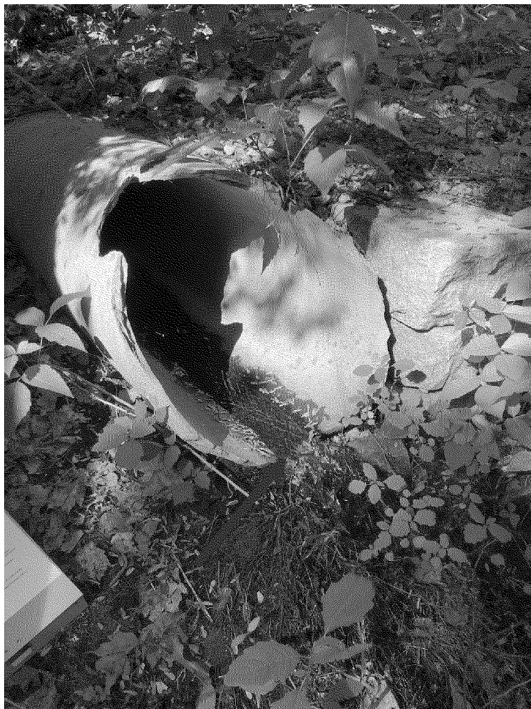
Renfrew (photo taken 5/24 at 08:48 AM): Outfall located on the northeast side of the Renfrew Street bridge over Bare Meadow Brook. Sample point is indicated by a red arrow.
