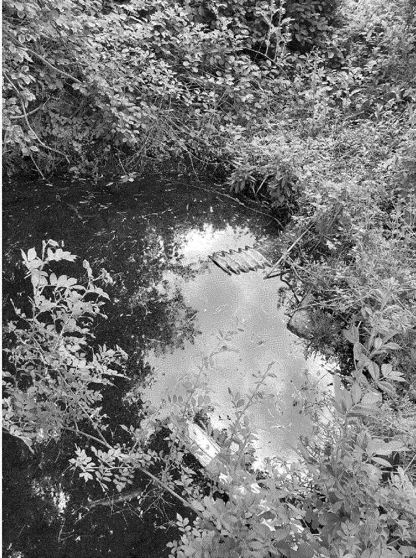
ECapitol (photo taken 5/24 at 14:45 PM): Outfall located at the corner of East Capitol Street and Marc Ave, adjacent to 47 East Capitol Street. The outfall is completely submerged. No sample was collected at this location.
