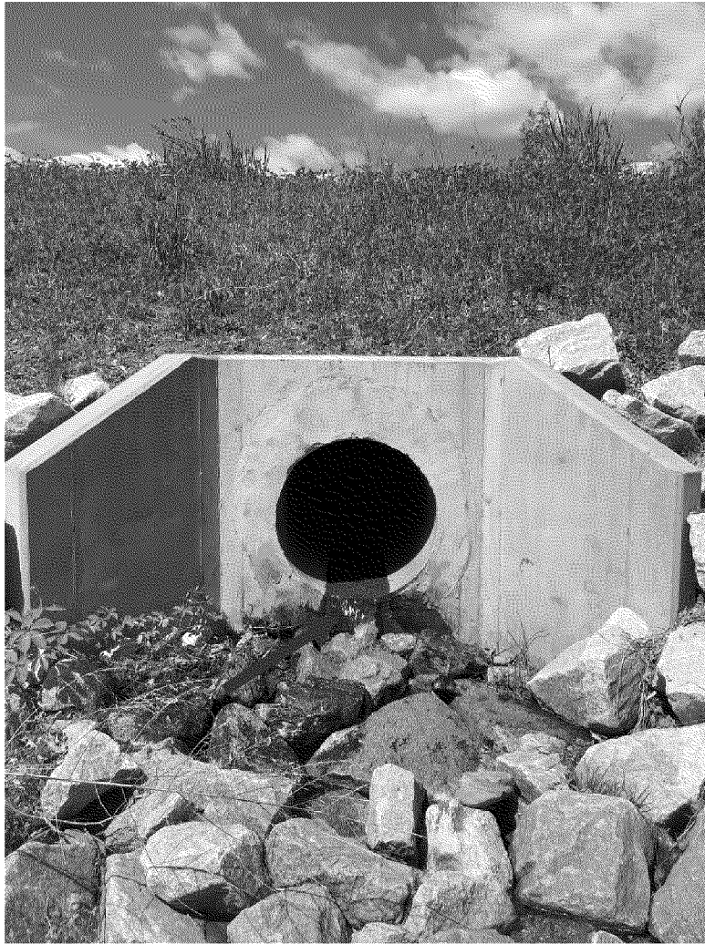
459MerrSt (photo taken 5/24 at 10:32 AM): Outfall located near 459 Merrimack Street flowing into the Merrimack River. Sample point is indicated by a red arrow.
